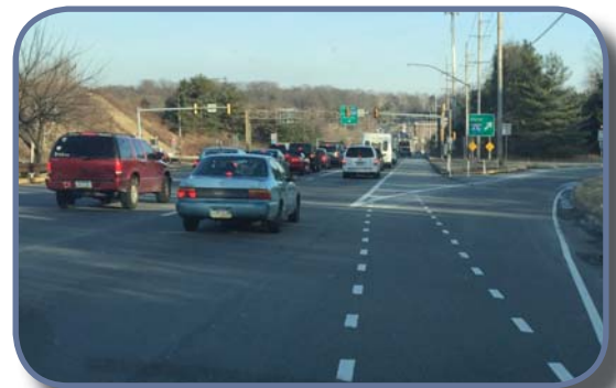
I-476 at PA-3: Merge with dashed lines across the right exit turn lane in the shoulder. Photo Credit: DVRPC
