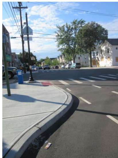
A curb extension
