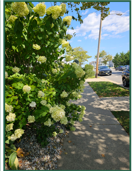
Figure 14. Vegetation encroaching into the sidewalk near 8th Avenue and B Street.
