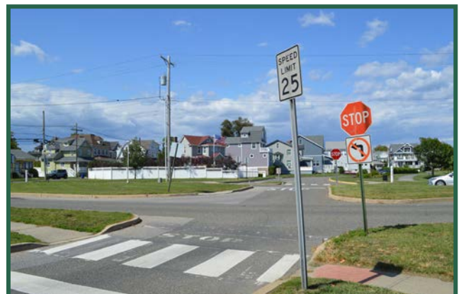
Figure 19. Looking north from S. Lake Dr., there is a stop control to enter the oval and again to continue straight or left.
