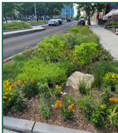
Figure 41. Curb extension in Newark.
