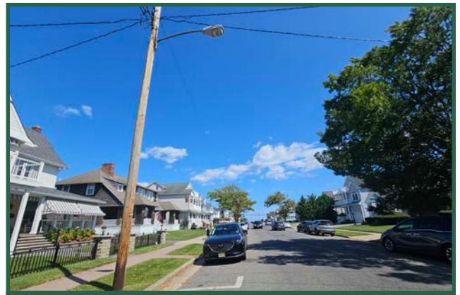
Figure 22. Overhead lighting, located mid-block.
