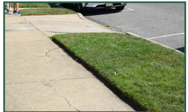
Figure 57. Cracked sidewalk.
