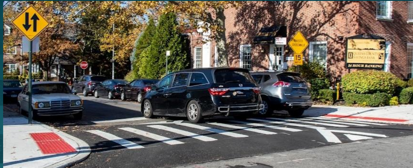
Example of raised pedestrian crosswalk
