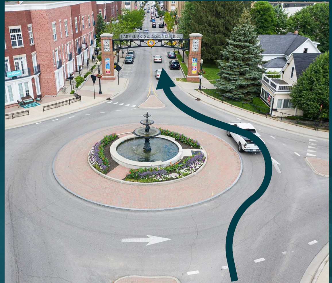
Roundabout geometry influences speed
