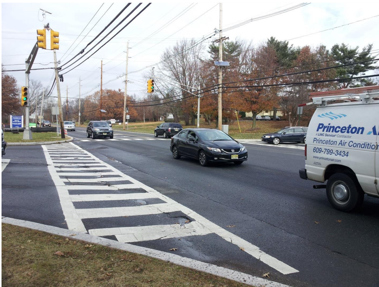
Figure 21: Crosswalk without signal and lacking ADA Compatibility, Montgomery, 11/22/2013
