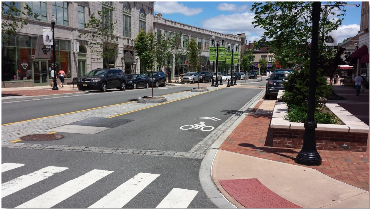
Figure 16: Sharrow, Pedestrian Bay, and Curb Cutout in Montclair Addresses Bike/Ped Safety, 6/6/2014
