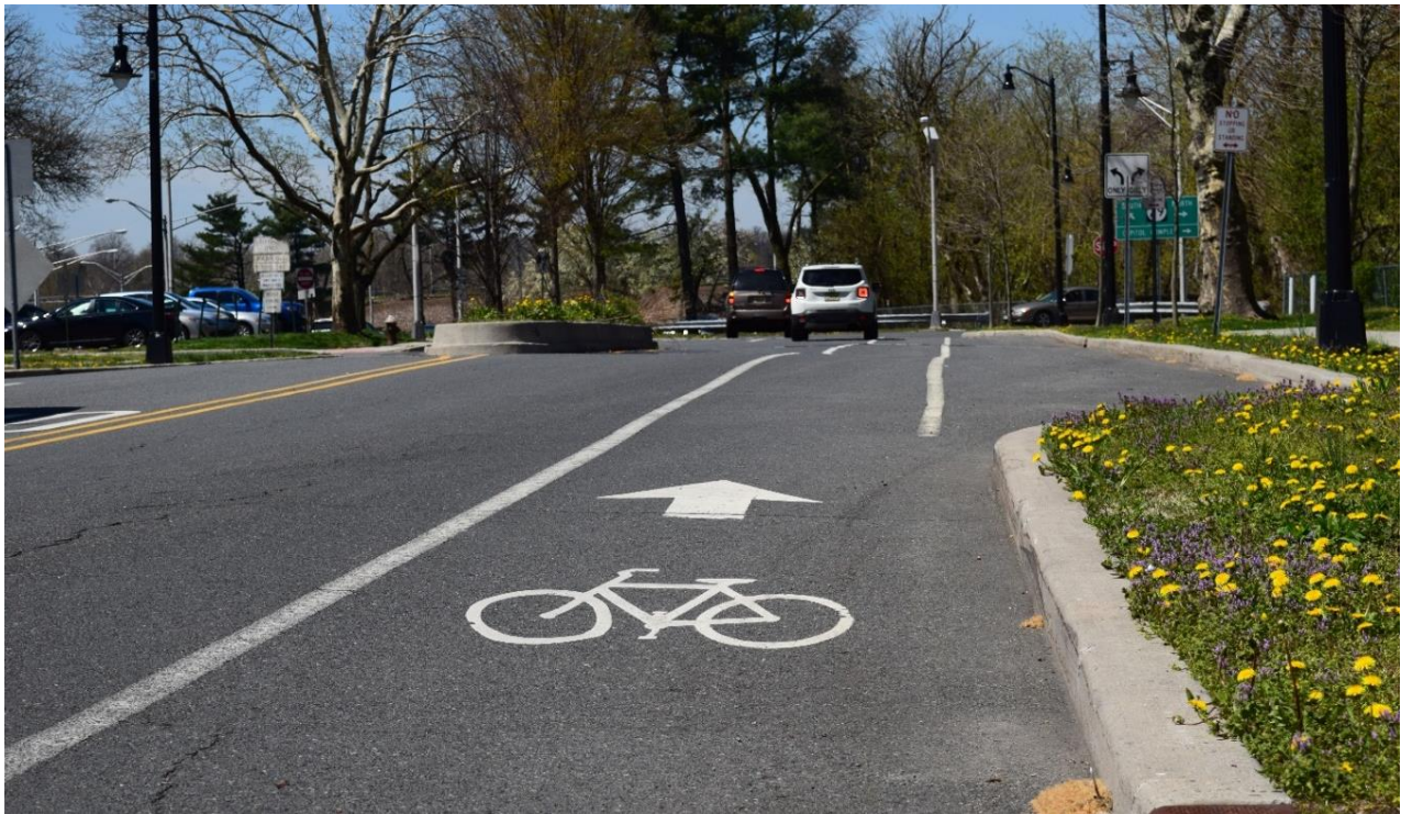
Figure 12. An image of a bicycle lane in Trenton, NJ. This is one of the many Complete Streets images included in the NJBPRC image repository.
