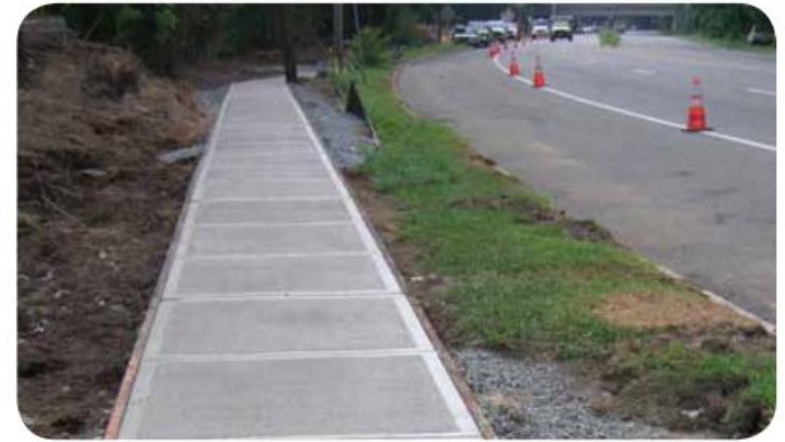
New sidewalk. Image: VTC
