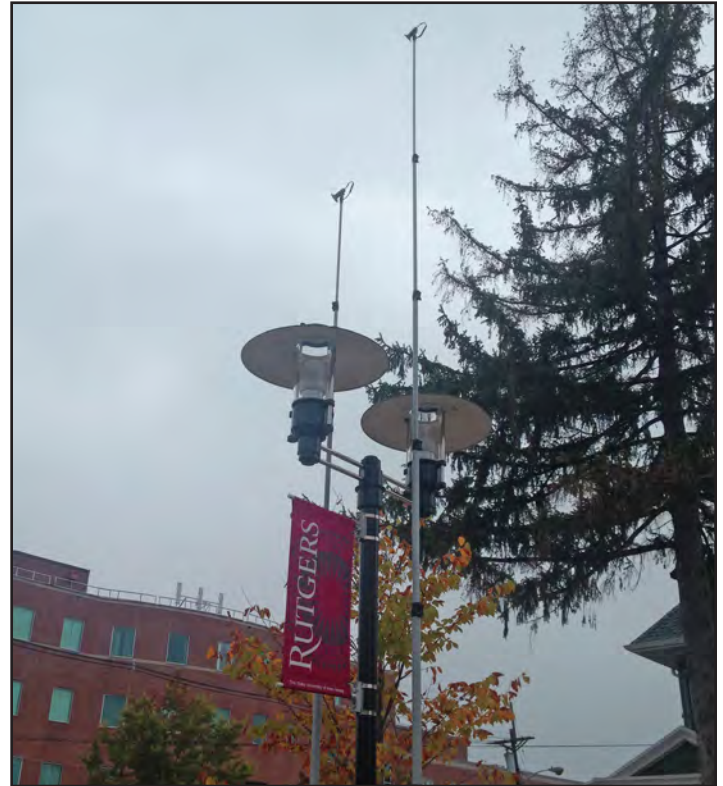
Figure 11. Video Camera Rig (Attached to Street Lighting)
