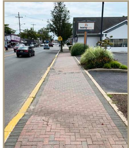
Figure 15. Likely non-compliant driveway ramp cross slopes on Main Street, between Fifth and Brinley Avenue.
