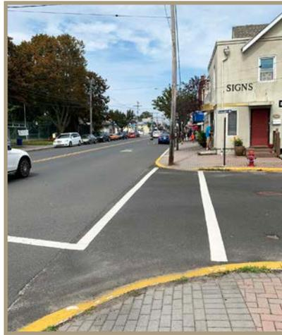
Figure 35. Curb ramps and standard crosswalks at the Monmouth Avenue intersection.
