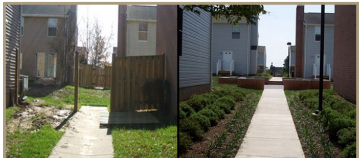
Figure 4. An apartment complex entrance before (left) and after (right) maintenance. Source: ICP Consulting
