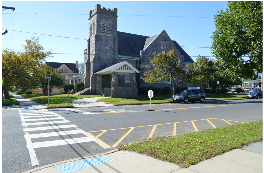
Figure 13. New high-visibility crosswalk, hatched no parking zone, and additional stop sign.
