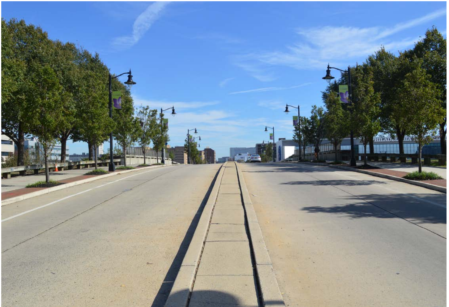
Figure 1. Dr. Martin Luther King Boulevard, Camden, New Jersey
