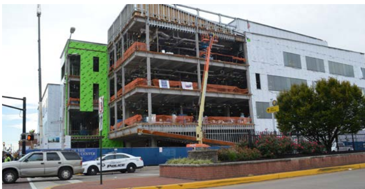
Figure 22. Construction in Camden
