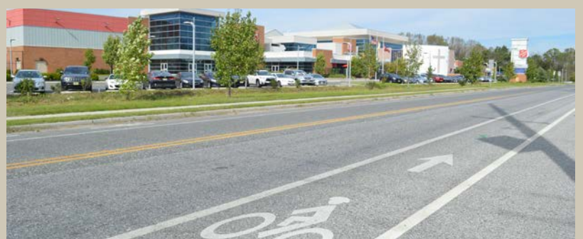
Figure 11. Bicycle lanes in front of the Kroc Community Center
