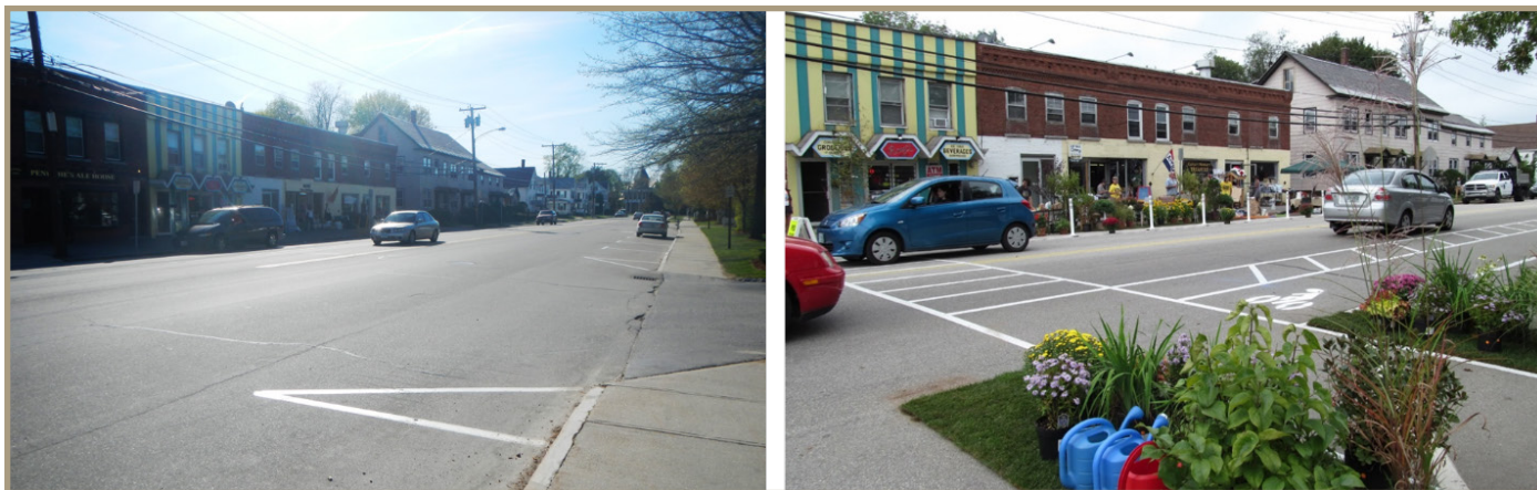
Figure 24. Complete Streets Transformation of a Wide Section of Roadway - Before (left) and After (right) (Source: Mari Brunner)
