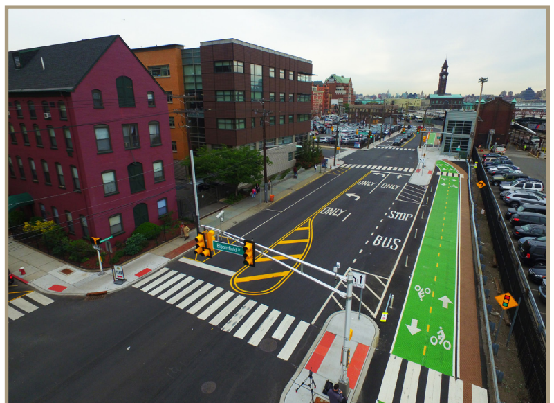
Figure 1. A Complete Street as seen in Hoboken, New Jersey (Source: The City of Hoboken)
