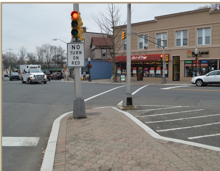
Figure 19. Crosswalk on southeast corner of plaza is not ADA-compliant and lacks pedestrian signals (looking south).
