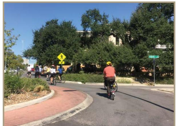
Figure 66. A permanent mini-roundabout with mountable curb in a neighborhood in Austin, TX. (Photo Credits: Global Street Design Guide)
