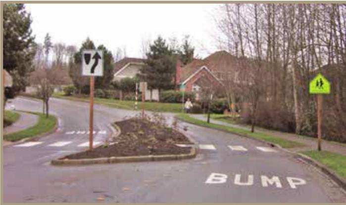
Figure 70. A 12 feet wide, 3 inches high speed hump installed on a crossing in Bellevue, WA (Photo Credits: City of Bellevue)
