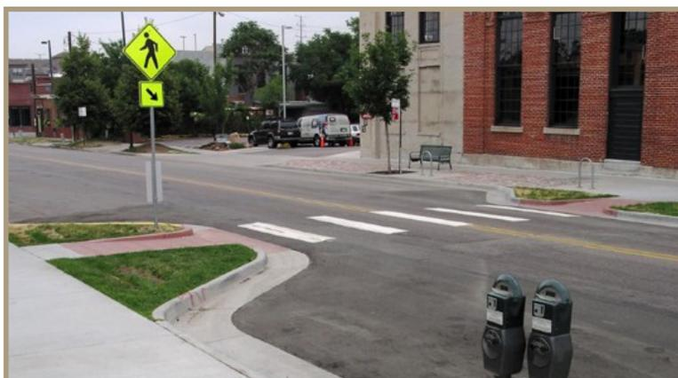
Figure 61. Traffic calming neckdown at a mid-block crossing. (Photo Credits: Deeprout Green Infrastructure)
