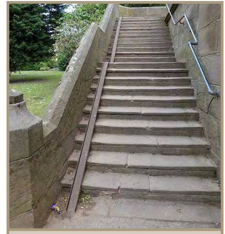
Figure 43. A wheeling ramp on the left side of the staircase. Photo: Oliver Dixon.
