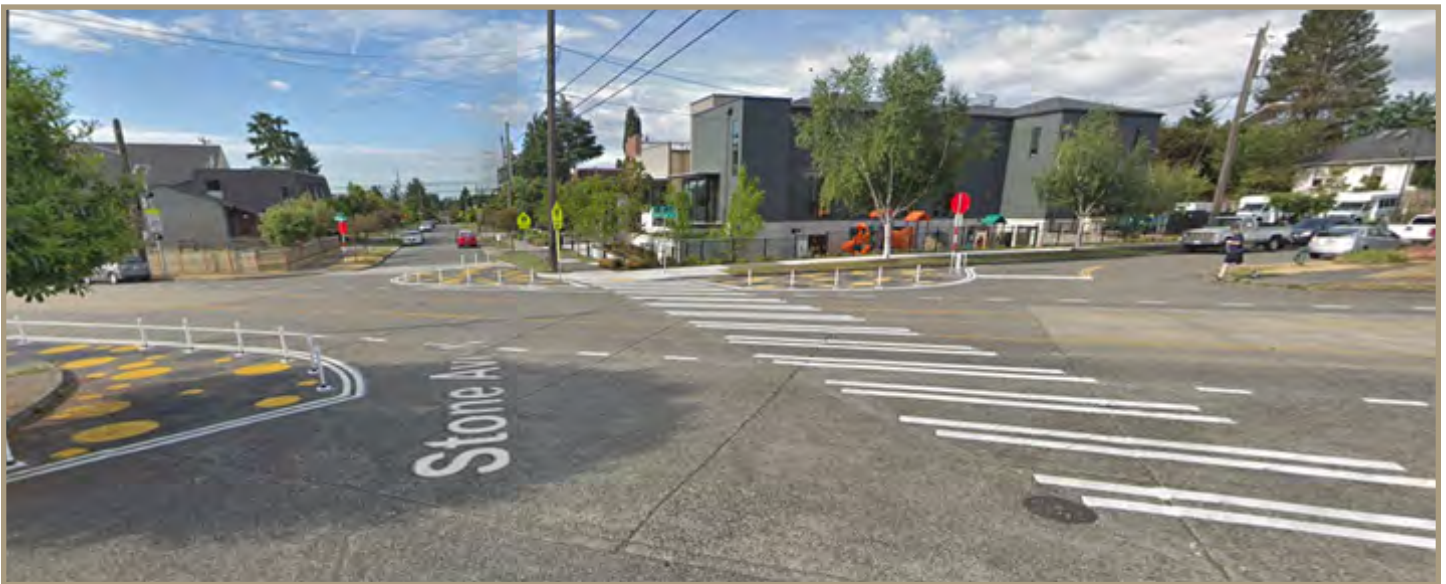
Figure 55. Curb extensions using plastic bollards and paint have been used in Seattle to realign confusing intersections, slow traffic, and add new pedestrian crossings.
