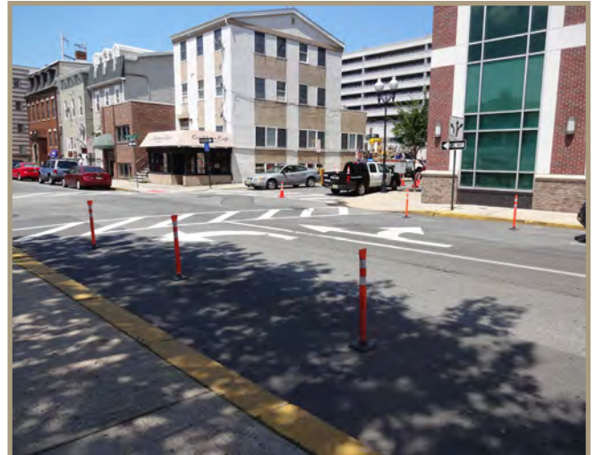
Figure 54. New Brunswick, NJ, uses plastic bollards to prevent illegal parking near intersections. After a successful trial at one intersection, the city has added them throughout the city.
