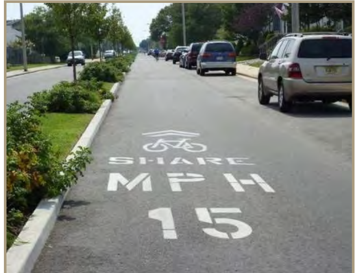
Figure 48. Pavement markings in Ocean City, New Jersey.
