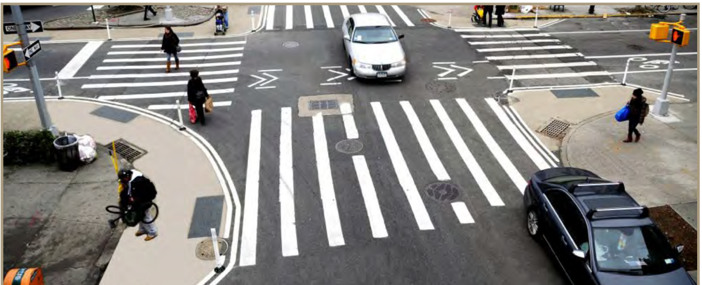
Figure 58. New York City has made extensive use of paint and plastic bollards to decrease turn radii at intersections throughout the city.
