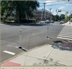
Figure 26. White plastic bollards to alter turning radius. New Brunswick, New Jersey.
