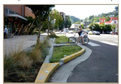
Figure 12. Green infrastructure used to narrow the roadway and provide a shorter crossing distance for pedestrians.
