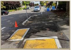
Figure 31. Sidewalk built using parking stops, Seattle, Washington.
