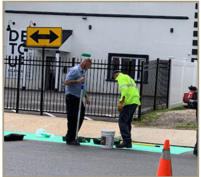
Figure 30. Red Bank municipal employees installing the demonstration project.
