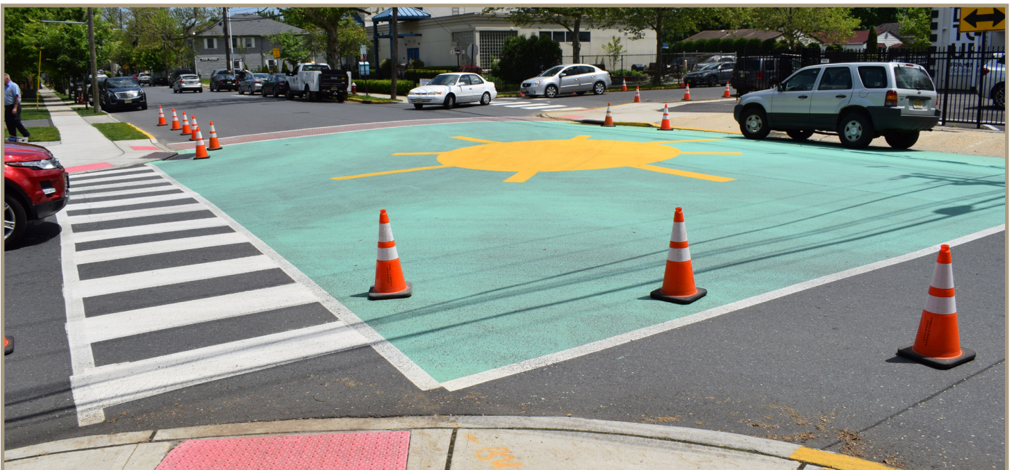
Figure 1. Intersection of Drs. James Parker Boulevard and South Bridge Street after project implementation.
