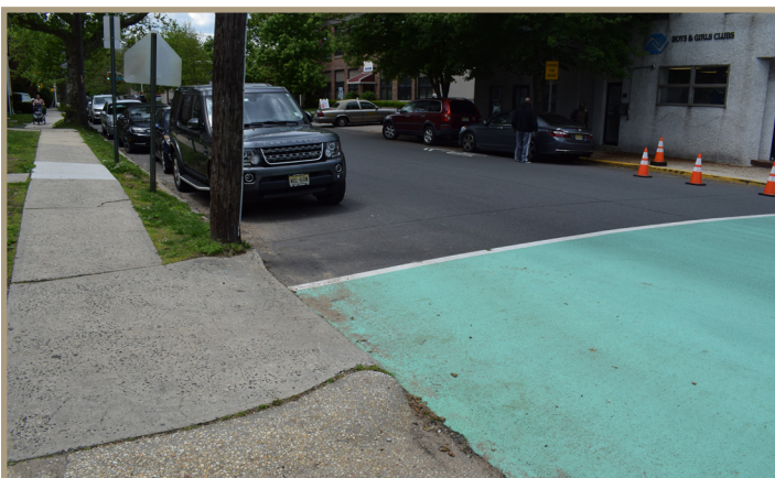
Figure 46. The telephone pole blocks the potential location of a curb ramp for a crosswalk.
