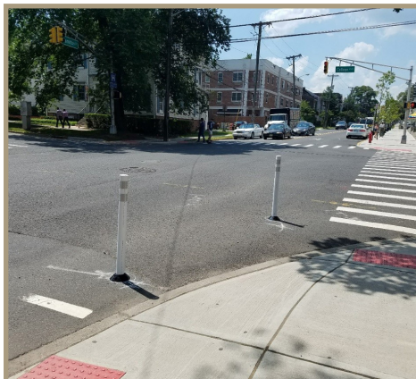
Figure 22. White plastic bollards to alter turning radius. New Brunswick, New Jersey.
