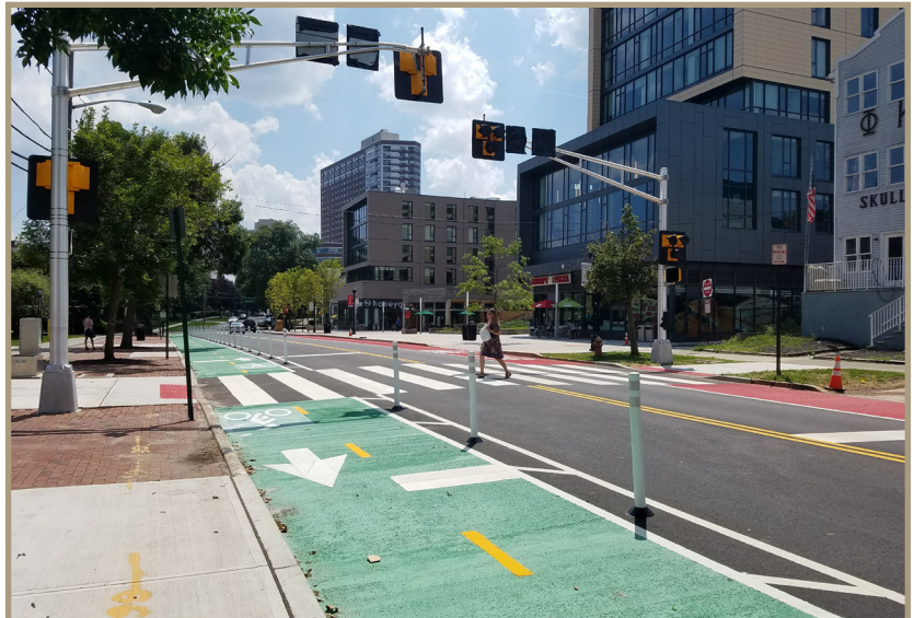
Figure 2. A complete street, as seen in New Brunswick, New Jersey. No two complete streets are alike, as they should always reflect the context of the street and the character of the community.
