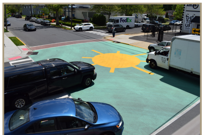
Figure 19. The offset design of the intersection makes it challenging for vehicles to navigate even without the presence of pedestrians. This photo was taken after the mural was painted, but before the cones were set in to limit the width of the travel lanes.
