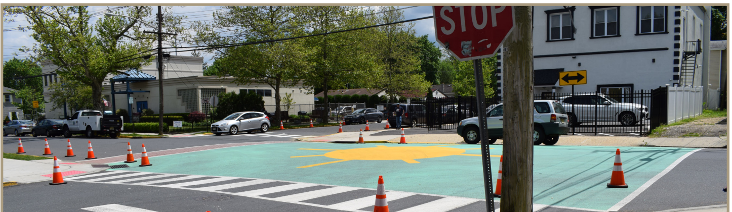
Figure 42. Traffic cone placement not only slows turning traffic, it also shortens the crosswalk distance.
