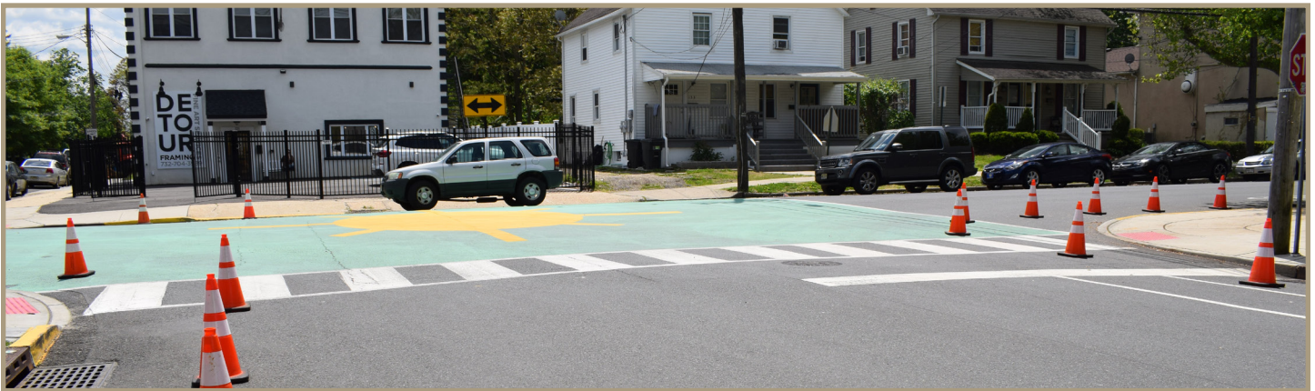
Figure 45. The telephone pole on the opposite side of Drs James Parker Boulevard blocks the potential location of a curb ramp for a crosswalk.
