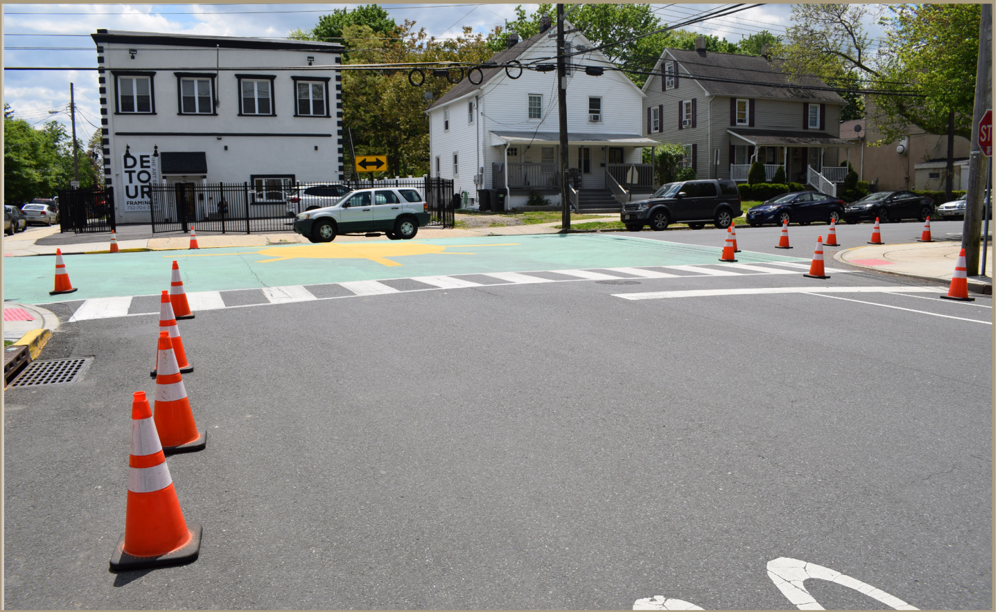
Figure 32. Traffic cones placed to temporarily extend the curb and slow turning traffic. Looking south on South Bridge Street.
