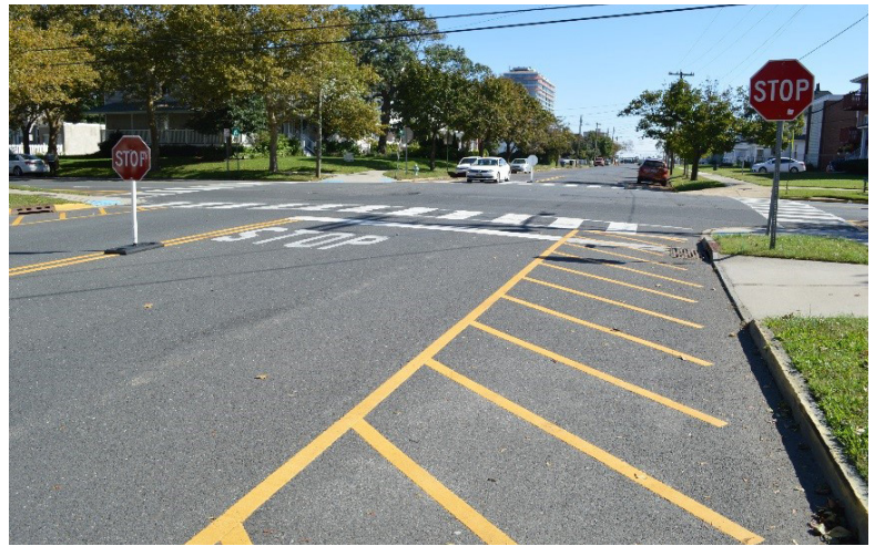
Figure 1. Portable stop sign added to supplement standard signage and pavement stencils in Asbury Park, NJ.
