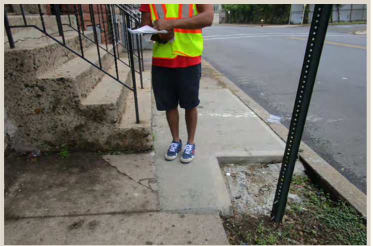
Figure 129. Signage and stairs create a narrow walkway.
