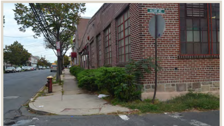
Figure 15. Building at corner of Brunswick and Hillside blocks sight lines for vehicles arriving at the stop sign.
