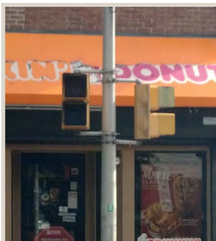
Figure 83. Non-functioning pedestrian signal
