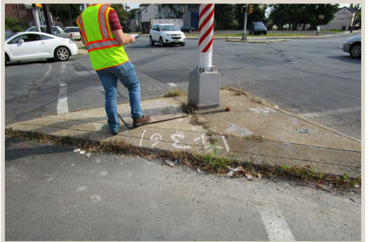
Figure 146. Missing ramps on pedestrian island.
