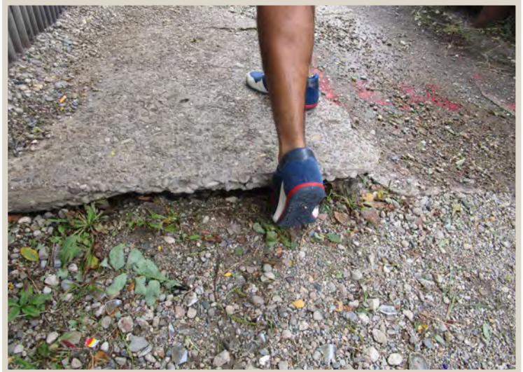
Figure 134. Sidewalks in extremely poor condition.
