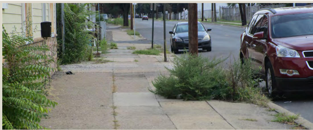
Figure 59. Cracked sidewalks and overgrown weeds.
