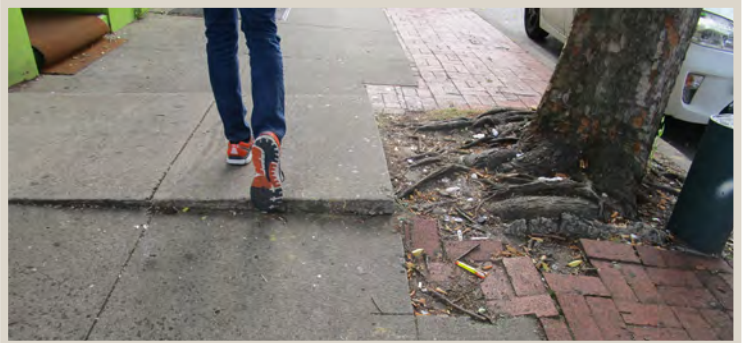
Figure 166. Raised sidewalk causes a tripping hazard.
