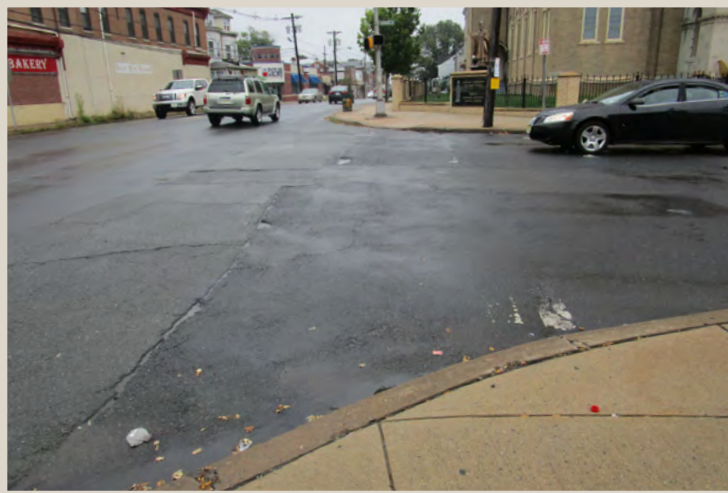
Figure 118. Severely faded crosswalk and stop lines.
