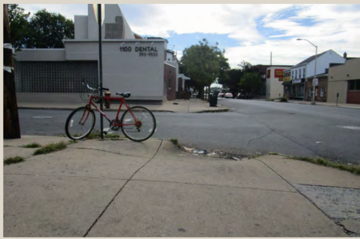
Figure 169. Steep ramp with litter.
