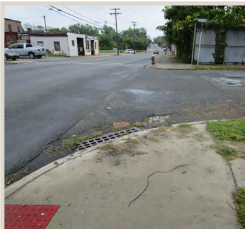
Figure 130. Missing curb ramps.
