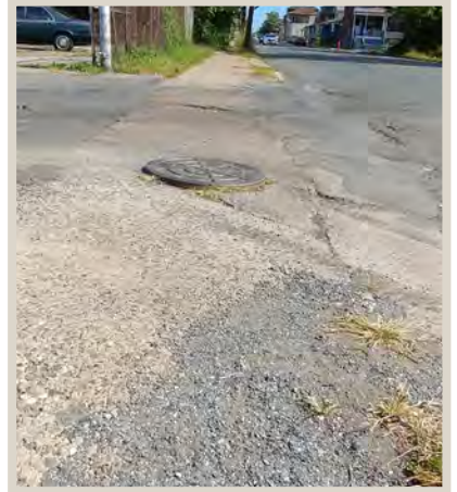
Figure 29. A sloping, uneven sidewalk.
