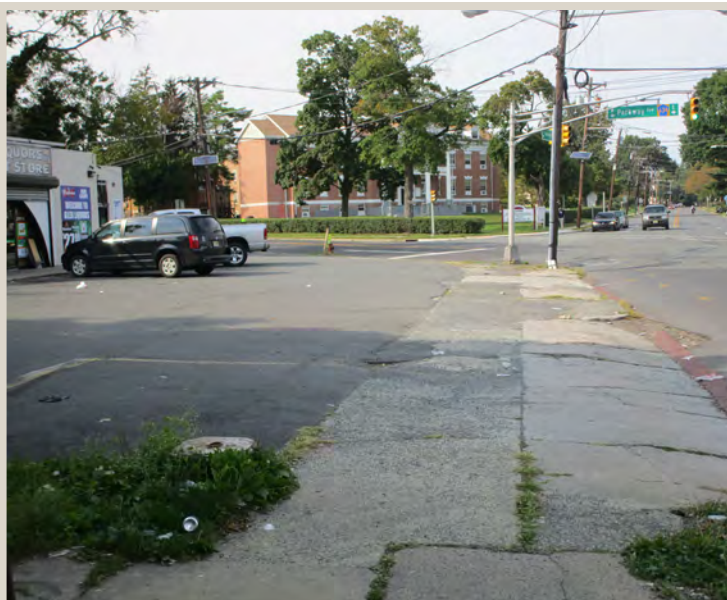
Figure 139. Continuous driveway access across sidewalk.
