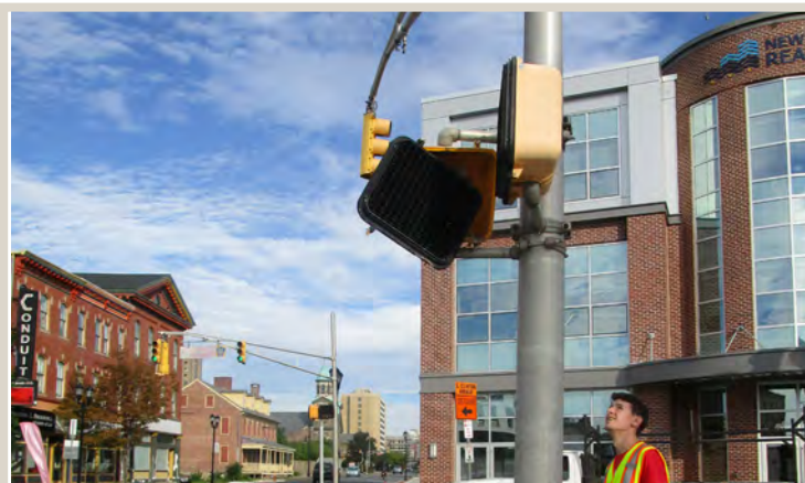
Figure 162. Non-operational pedestrian signal.
