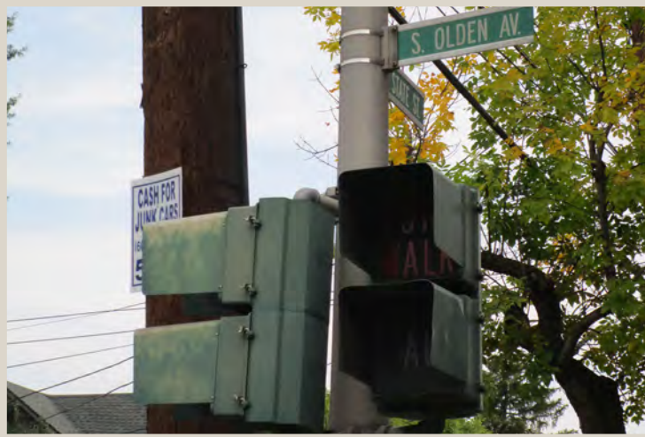
Figure 62. Dim and outdated pedestrian crossing signals.
