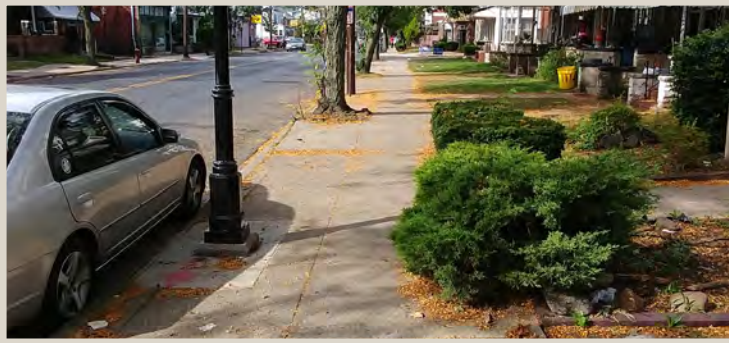
Figure 85. Five-foot wide sidewalks in generally good condition.
