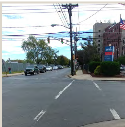
Figure 82. Faded crosswalks near hospital.
