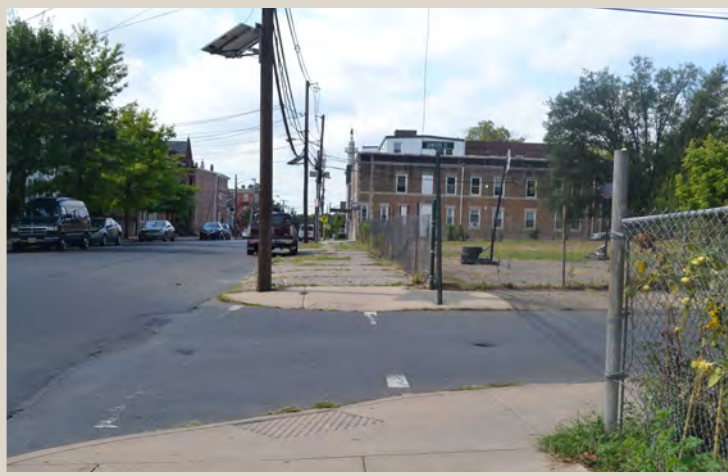
Figure 20. Brunswick Avenue and Sanford Street. Sidewalk in front of vacant property is in especially poor condition.
