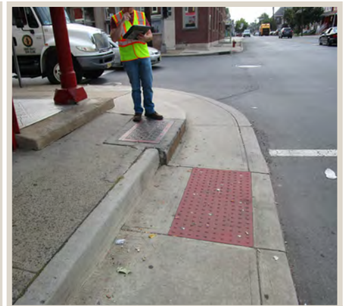
Figure 65. Challenging curb design.
