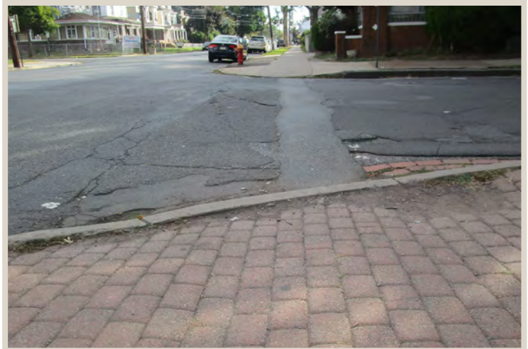
Figure 98. Missing crosswalk and non-compliant curb ramps.
