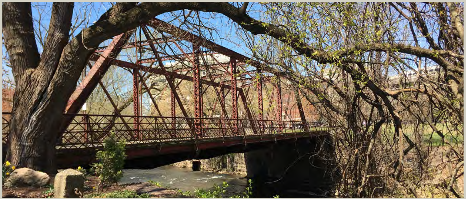
Figure 4. Jackson Street Bridge in Mill Hill Park, Trenton, New Jersey.
