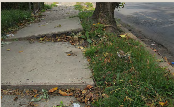
Figure 147. Roots have lifted the sidewalk into stairs.
