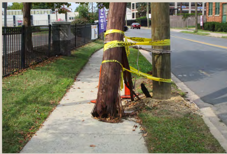
Figure 149. Haphazard utility pole work.
