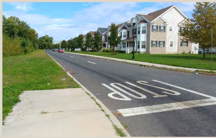
Figure 37. Improper white center striping along Dunham Street indicates that this roadway may be privately owned and maintained.
