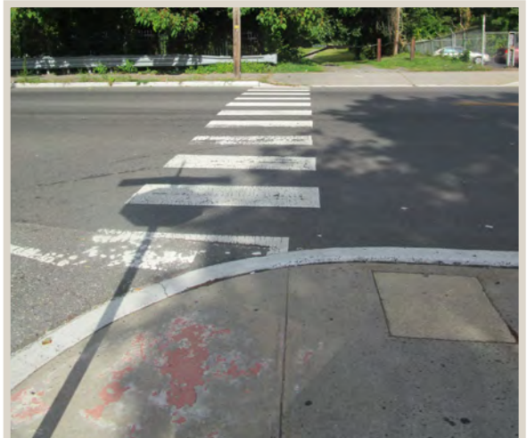
Figure 42. Continental crosswalk with faded ramps.
