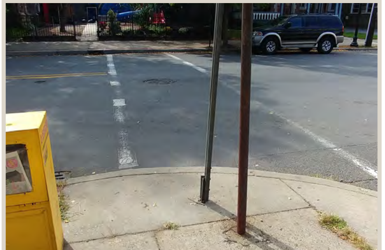
Figure 103. Missing curb ramps.
