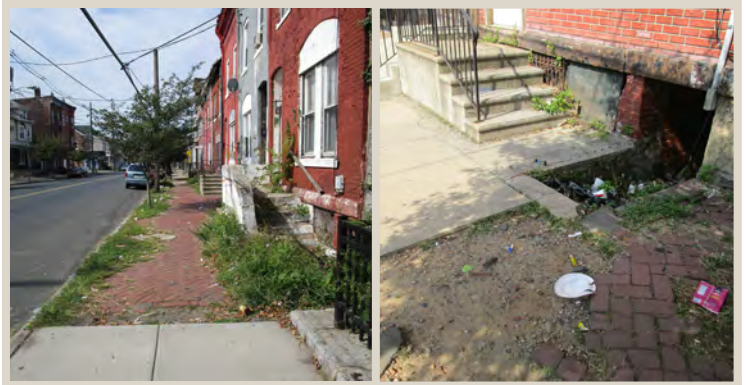
Figure 75. Gaps between varying sidewalk materials.
