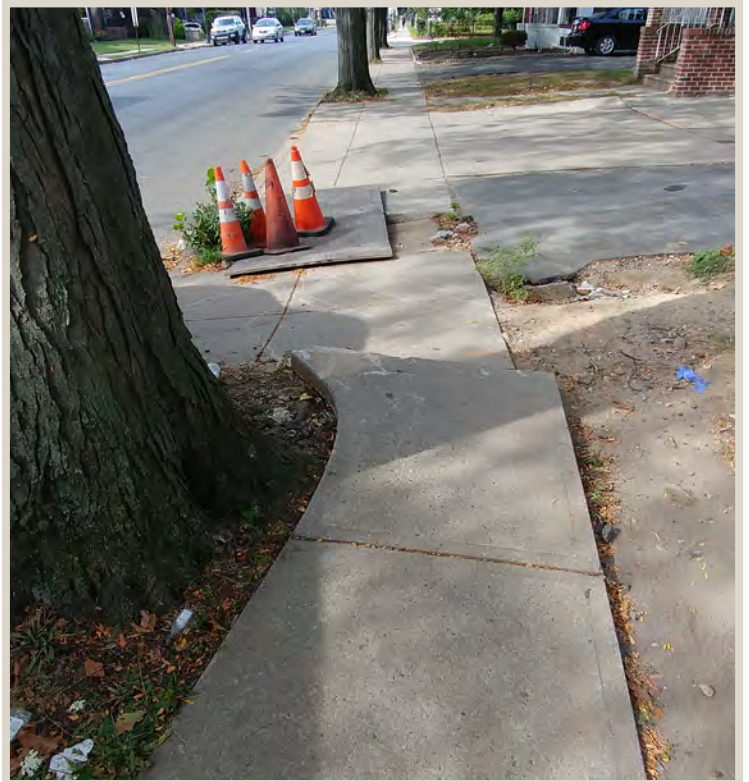
Figure 89. Tree-lifted sidewalk creates a barrier for some pedestrians.
