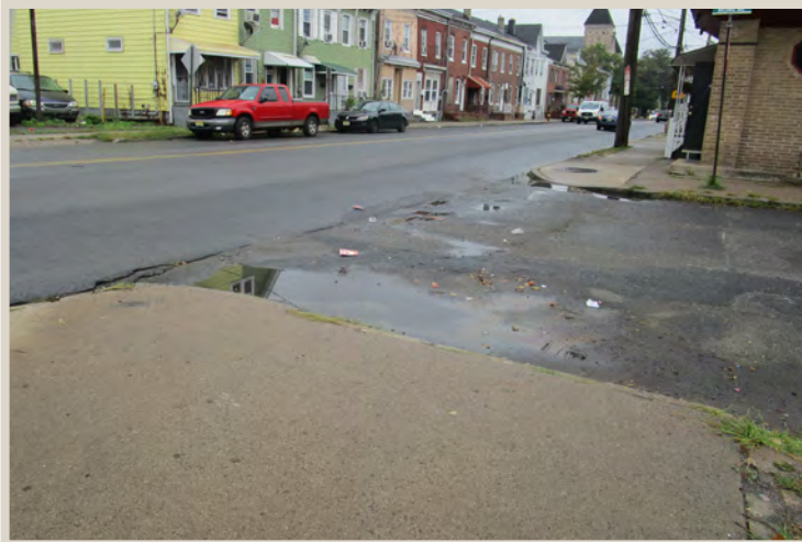
Figure 124. Missing crosswalk and non-compliant ramps.
