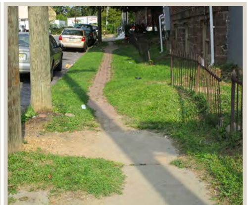
Figure 156. Sidewalk in poor condition.
