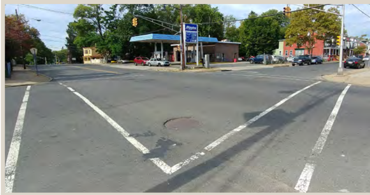
Figure 50. Intersection lacks pedestrian signals and ADA ramps.
