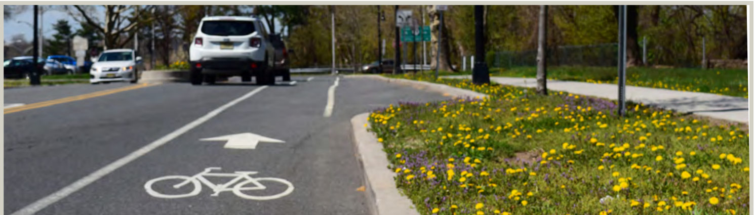
Figure 2. A Complete Street with bicycle lanes and curb bump-outs in Trenton, New Jersey.
