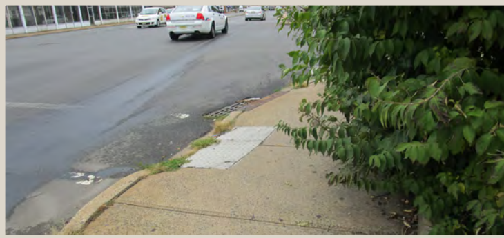
Figure 115. Non-compliant ramp with a bush blocking visibility.
