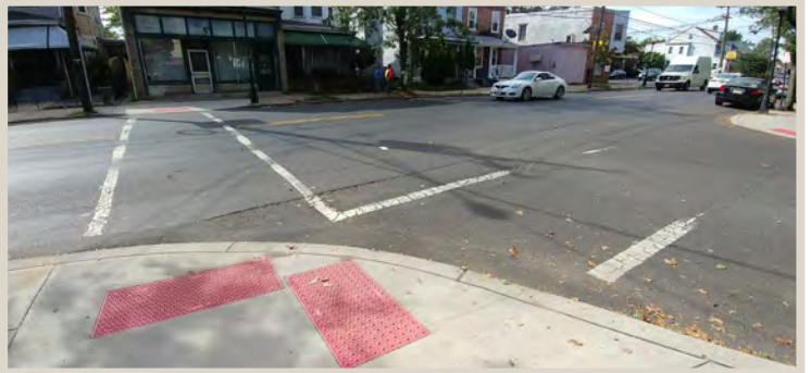
Figure 86. Faded crosswalk at Cuyler Avenue intersection.
