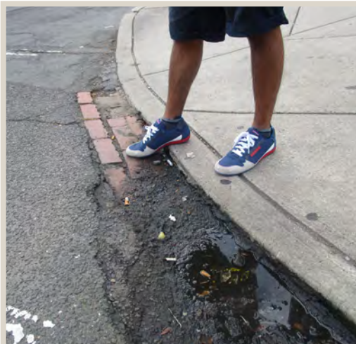
Figure 105. Compromised curb ramp.
