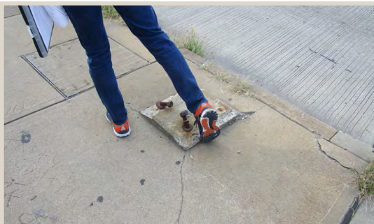
Figure 161. Tripping hazard along the sidewalk.
