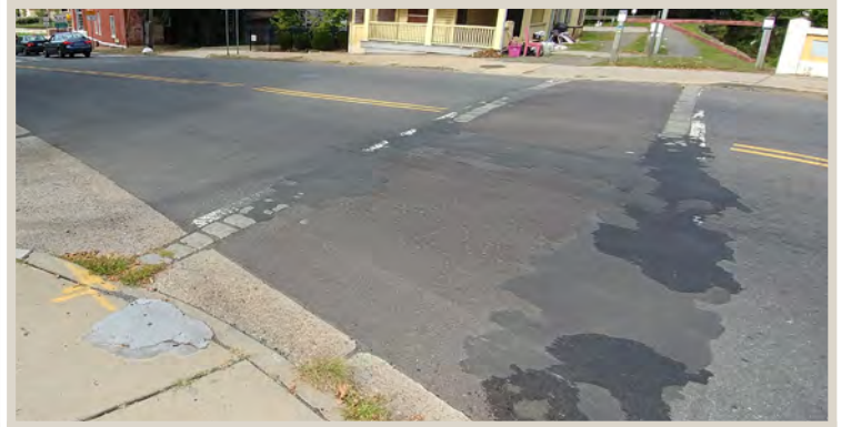
Figure 51. Asphalt-covered pavers along crosswalk.
