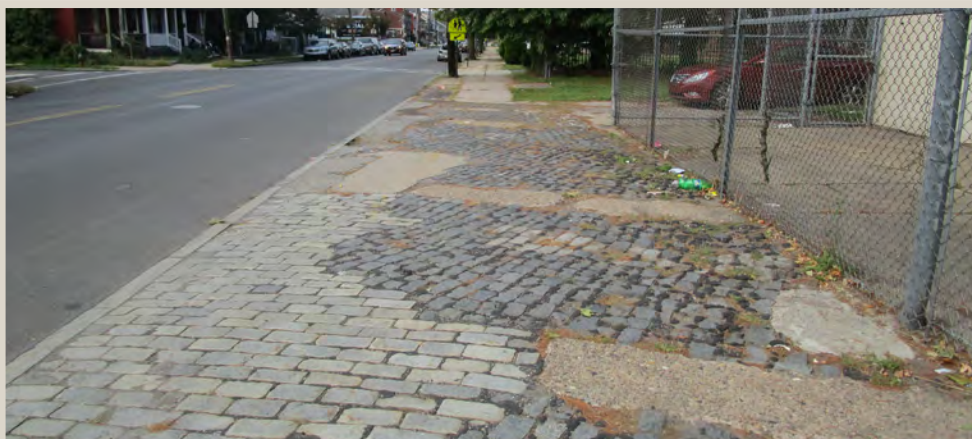
Figure 68. Uneven brickwork along East State Street.
