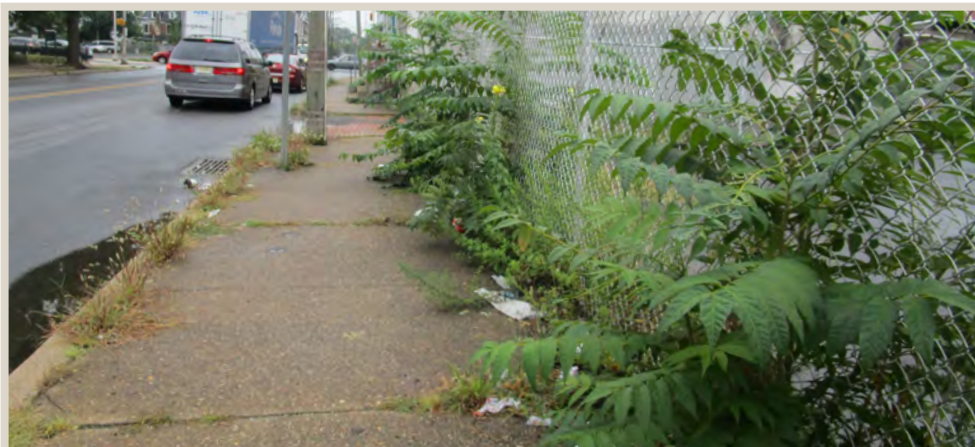
Figure 126. Overgrown brush blocking portions of the sidewalk.
