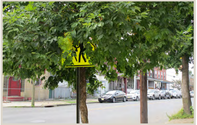
Figure 67. Mid-block crosswalk sign covered by overgrown tree.
