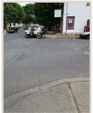
Figure 60. Missing curb ramps.
