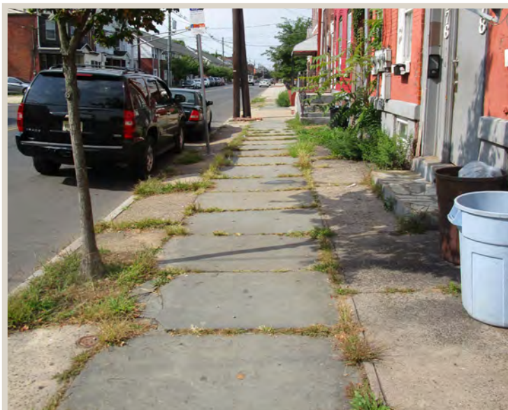
Figure 73. Vegetation growing between sidewalk panels.
