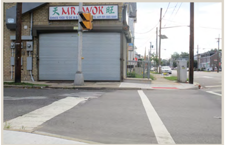
Figure 170. Misaligned pedestrian signal.
