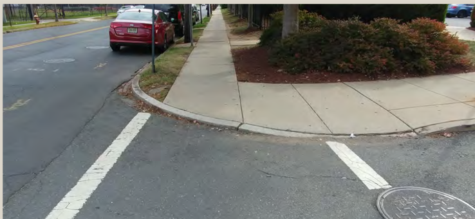
Figure 91. Non-compliant ADA ramps.
