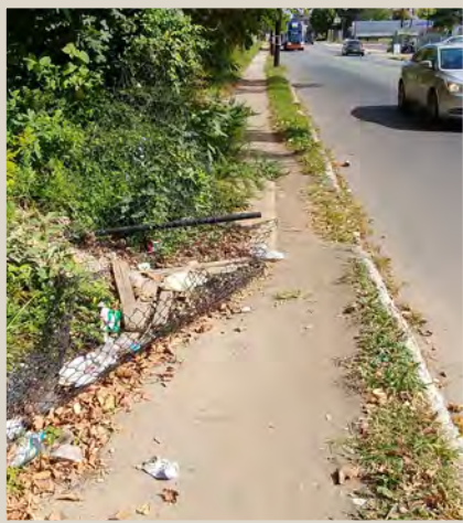
Figure 31. Fallen fence, litter and overgrown vegetation.
