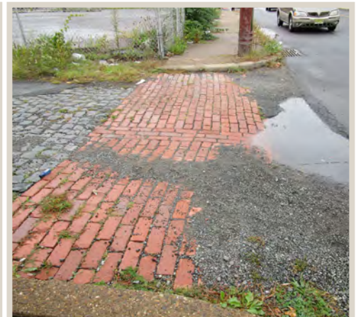
Figure 127. Missing curb ramps.
