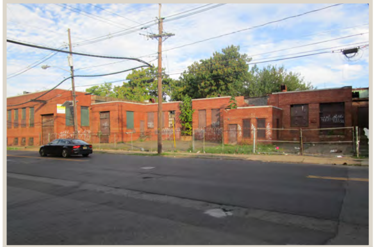
Figure 112. Vacant buildings are common in this section.
