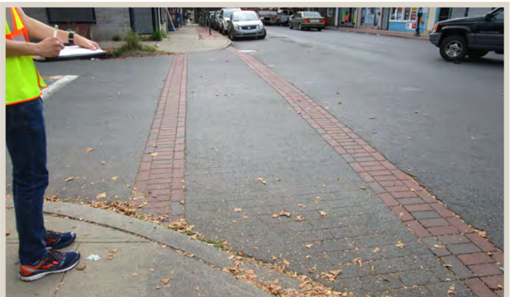
Figure 168. Crosswalk outlined in brick.
