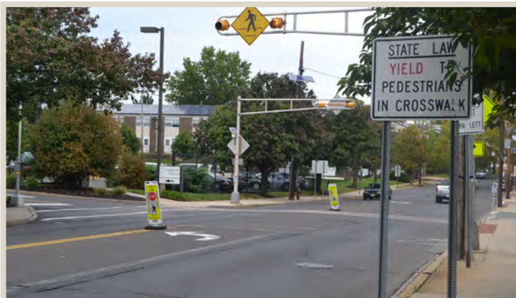
Figure 14. Crosswalk and pedestrian crossings signs by Capital Health Regional Medical Center.
