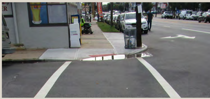
Figure 171. Water pooling at bottom of ramp.
