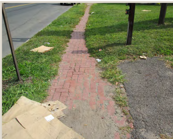
Figure 72. Sidewalk narrows and nearly disappears.
