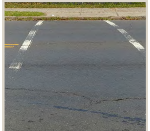
Figure 92. Faded crosswalk.
