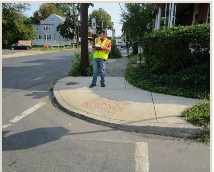
Figure 140. Large gap between bottom of ramp and roadway.
