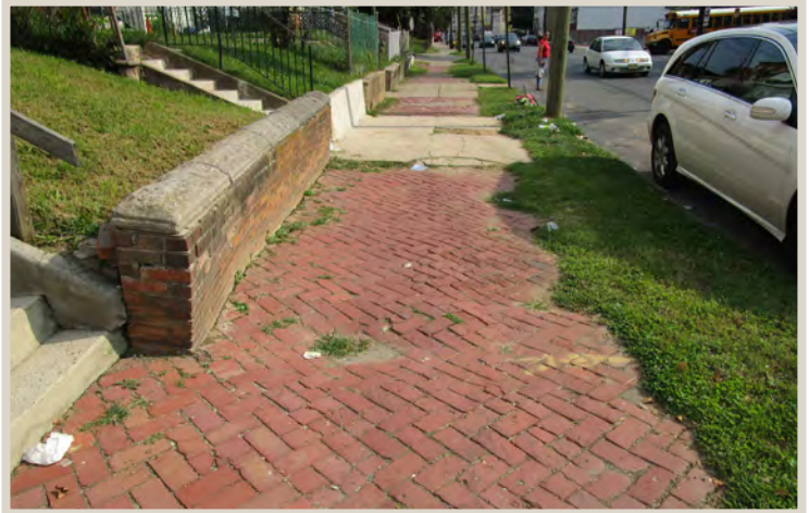
Figure 154. Sidewalk in poor condition.
