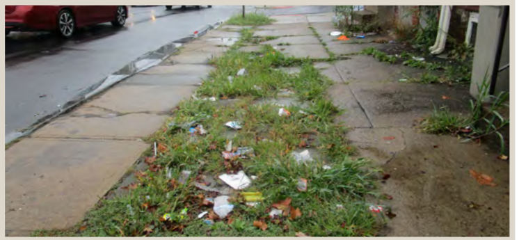
Figure 116. Missing sidewalk with litter.
