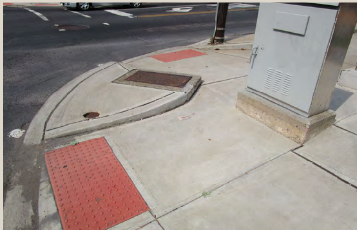
Figure 79. Retrofitted curb ramps at the Chambers Street intersection.
