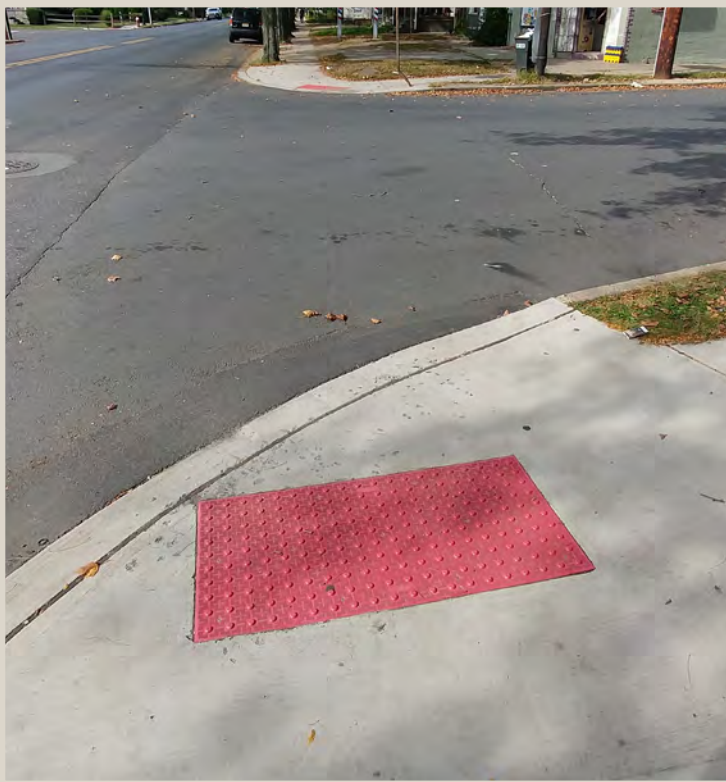
Figure 88. ADA compliant ramps, but missing crosswalks.
