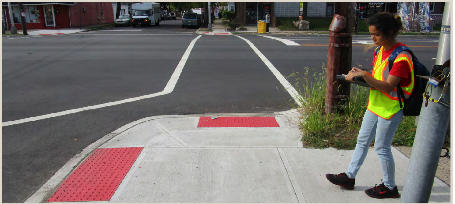
Figure 174. Sidewalks and ramps in excellent condition.
