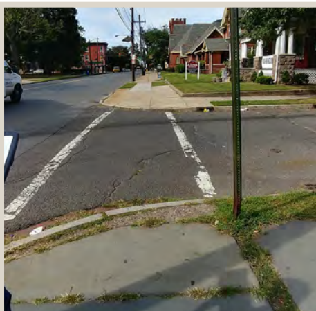
Figure 99. Missing curb ramps.
