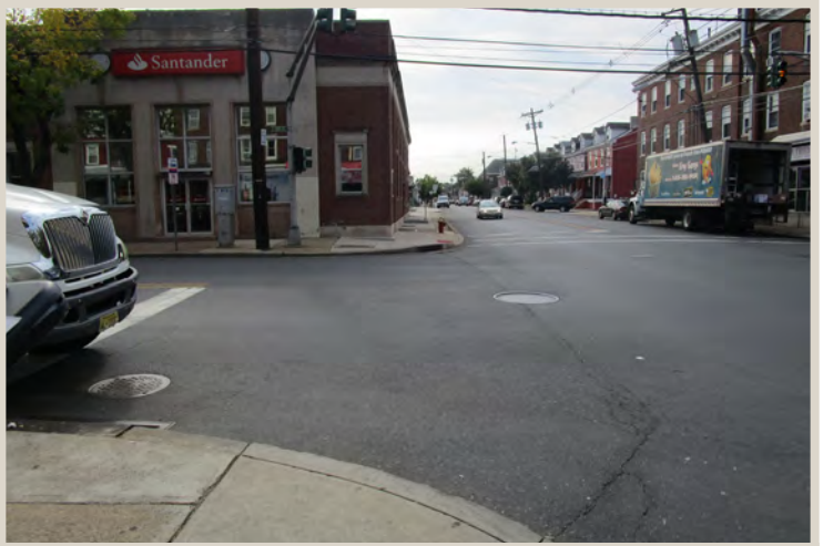
Figure 63. Missing crosswalk at North Olden Avenue intersection.
