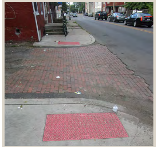
Figure 46. Small brick alley may create challenges for wheeled mobility devices.
