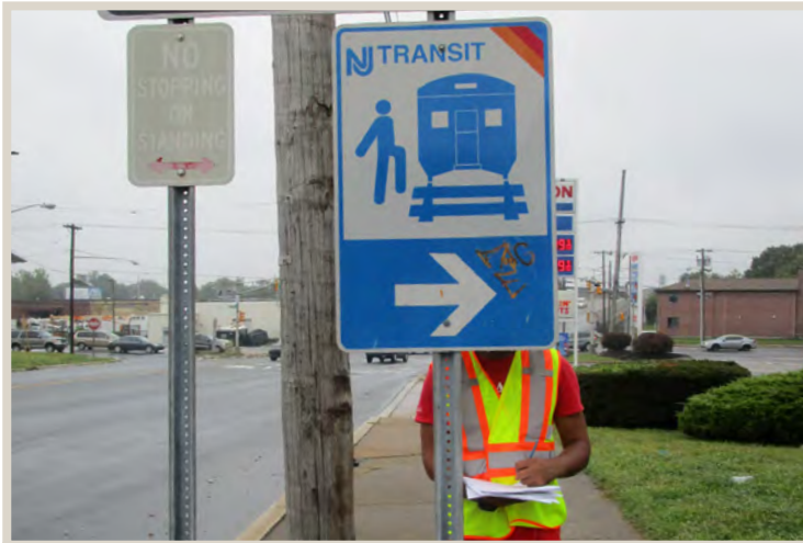
Figure 121. Faded and low-set signage.
