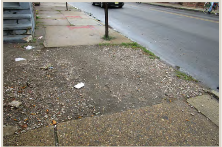
Figure 125. Sidewalk reduced to dirt and gravel.
