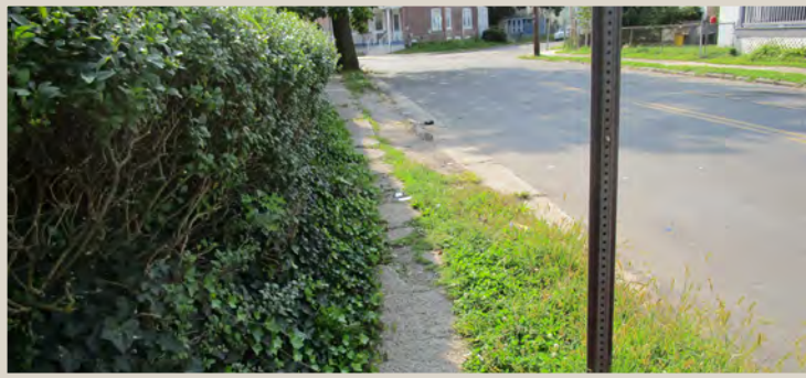
Figure 141. Overgrown plants blocking sidewalk.
