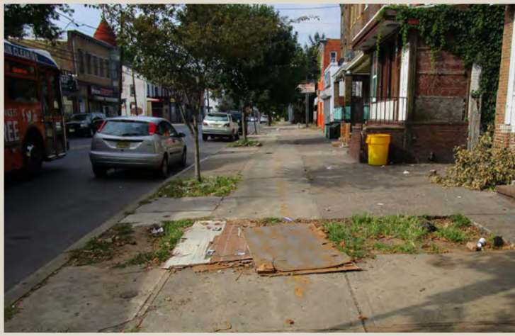
Figure 66. Missing sidewalk with makeshift bridge.
