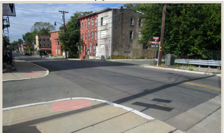
Figure 43. Missing crosswalks and faded ramps at the Church Street intersection.
