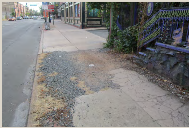
Figure 111. Sidewalk reduced to gravel.
