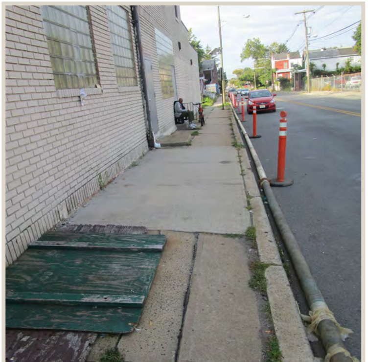
Figure 27. Steps making part of the sidewalk unusable.
