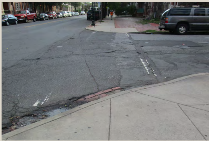
Figure 106. Faded crosswalks and non-compliant ramps.
