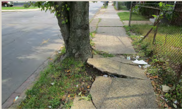
Figure 179. Dangerously uneven sidewalks along Pennington Avenue.
