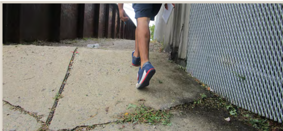
Figure 135. Steep incline along cracked sidewalks.
