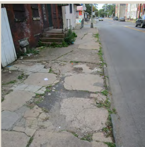
Figure 47. Significantly deteriorated sidewalk conditions.
