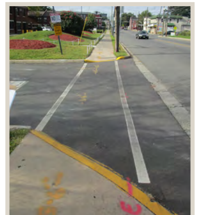
Figure 39. Non-compliant ramps.
