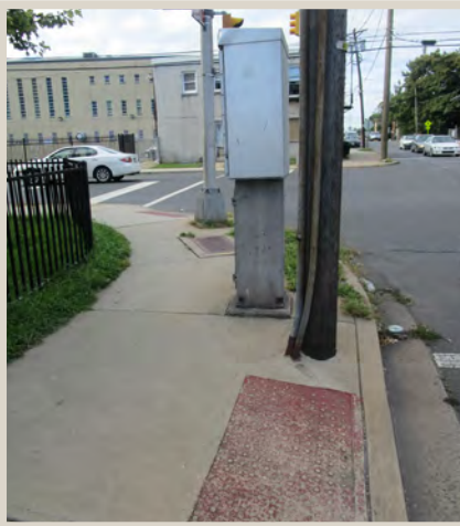
Figure 40. Electronic cabinet blocking pedestrians from drivers' sight.
