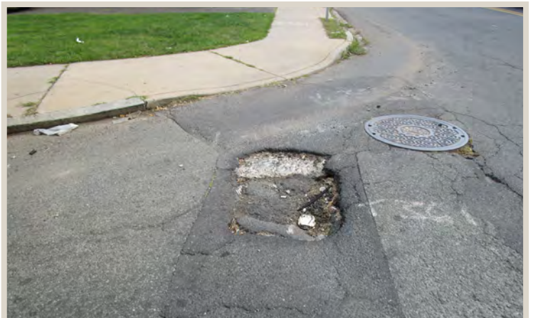
Figure 148. Asphalt near crosswalk in poor condition.
