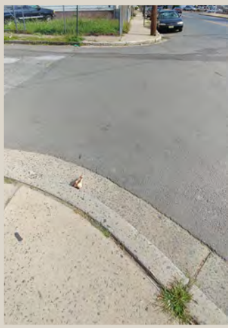
Figure 36. No ramps or crosswalks.
