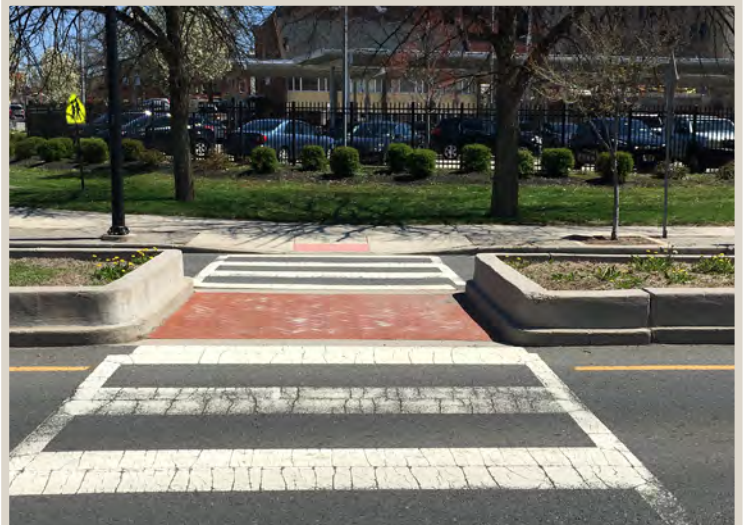
Figure 178. A pedestrian refuge located along S Warren Street.
