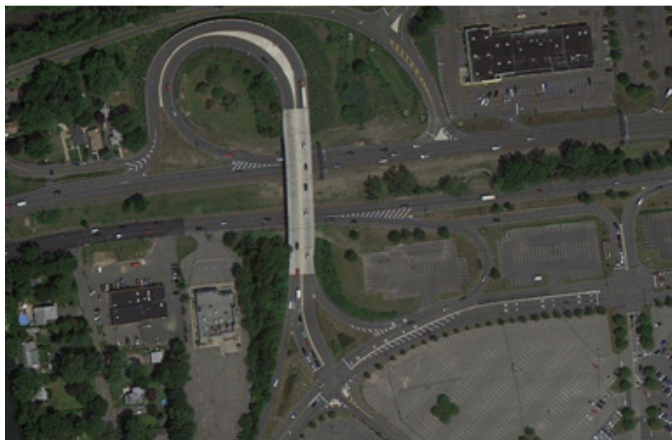
Figure 10: Overhead view of area pictured in Figure 9.
