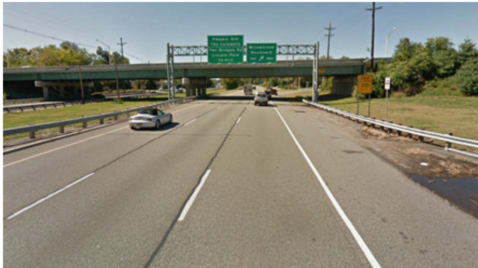
Figure 9: Highway 46, by Willowbrook Mall, in Wayne Township, Passaic County. Crash 55.
