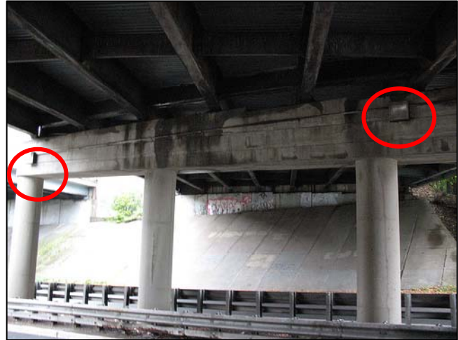
Figure 6. Typical roadway interchange lighting may not illuminate the pedestrian space. Pleasant Valley Way at I-280, West Orange, New Jersey.
