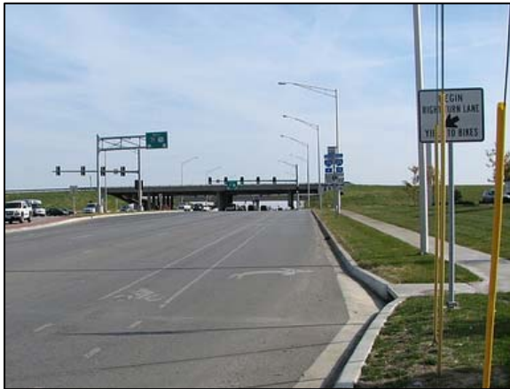
Figure 15. Yield to bikes sign at beginning of right turn lane to on-ramp. Barry Road at I-29, Kansas City, Missouri. Photographer: Eric Rogers
