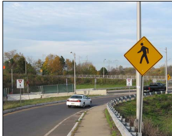
Figure 16. Pedestrian crossing warning sign in advance of a crosswalk on a highway exit ramp. Route 18 at Route 27, New Brunswick, New Jersey.
