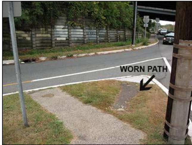
Figure 9. Worn path indicates pedestrians prefer to cross ramp parallel to roadway. Pleasant Valley Way at I-280, West Orange, New Jersey.
