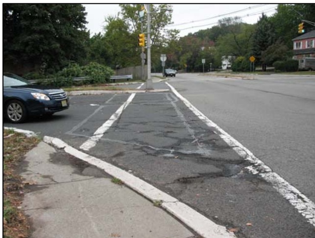
Figure 10. Lengthy crossing distance. Pleasant Valley Way at I-280, West Orange, New Jersey.
