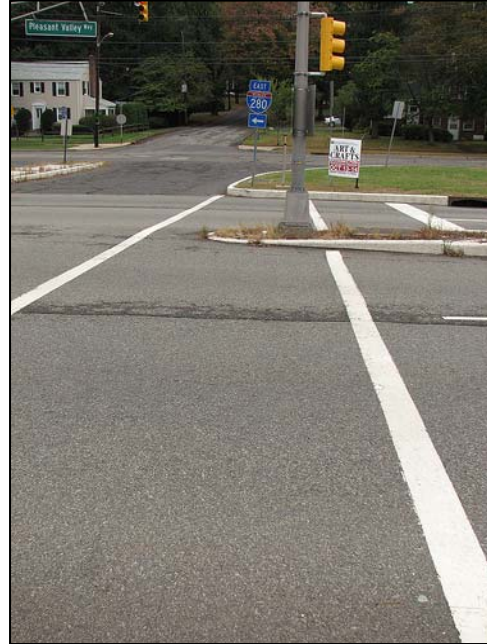
Figure 12. Striped crosswalk at I-280 ramp terminus and Pleasant Valley Way, West Orange, New Jersey.
