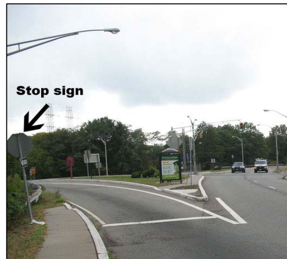
Figure 18. Ramp terminal with stop sign and an unmarked pedestrian crossing in advance of the stop sign. I-280 and Pleasant Valley Way, West Orange, New Jersey.
