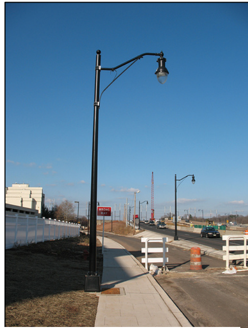
Figure 13. Lighting on Rt. 18 at Rt. 27. New Brunswick, New Jersey.
