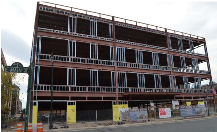
Figure 17. Somerville Commons, seen under construction on Main Street
