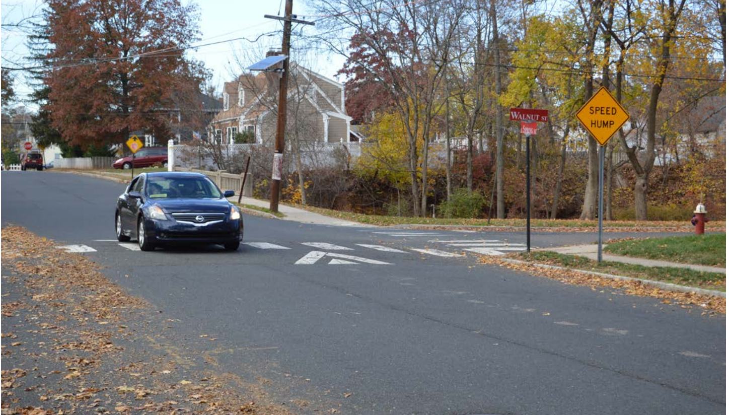
Figure 23. Speed humps combined with crosswalks work to calm traffic and increase pedestrian safety at some residential intersections
