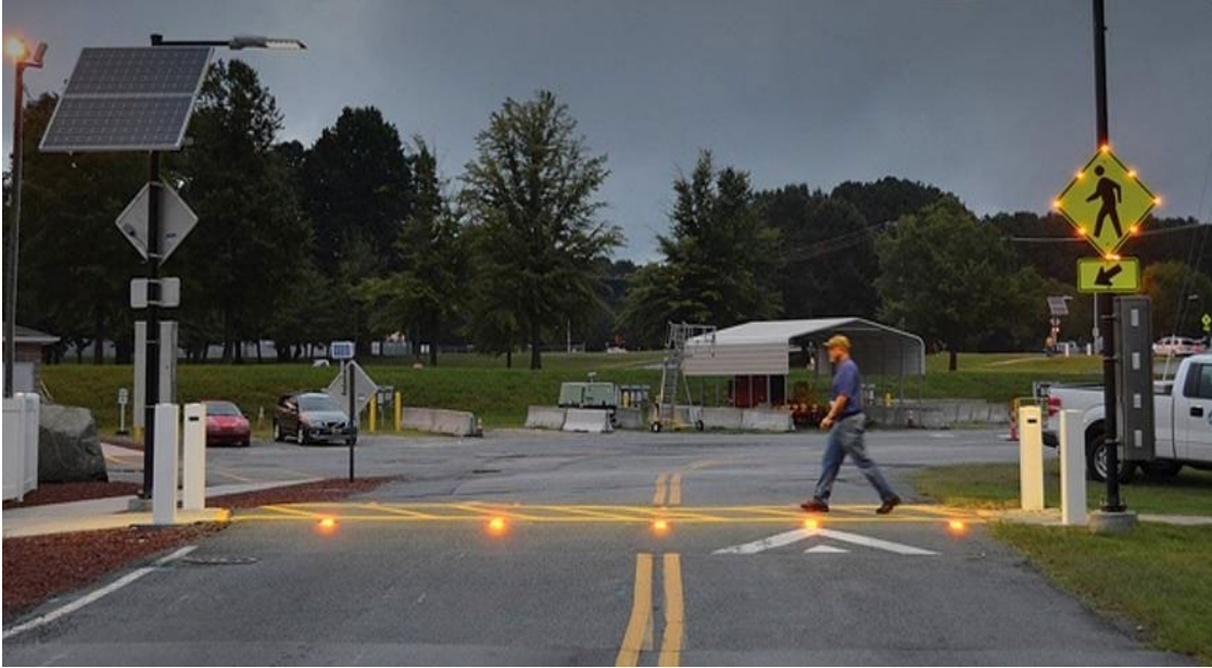
Figure 16. An in-pavement flashing light system (TAPCO, 2022)
