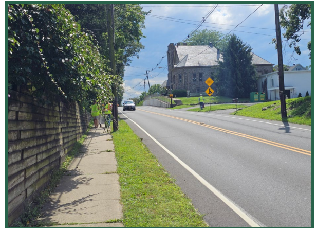
Figure 17. Missing sidewalk on west side of roadway north of Washington Drive.
