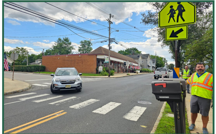
Figure 22. The Whitehouse Avenue crosswalk has high visibility striping and warning signage, but no curb ramps.
