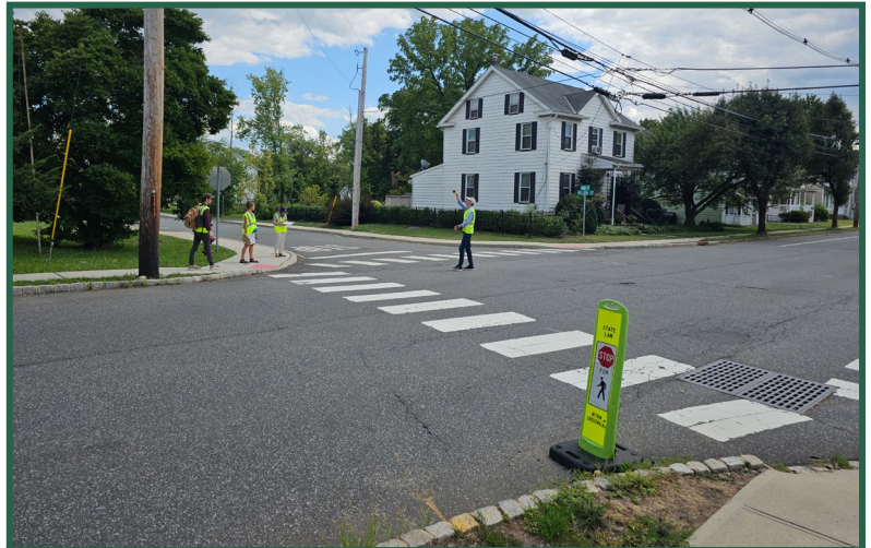
Figure 50. Nelson Street intersection, looking east.
