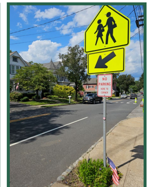
Figure 27. Striping continues into "no parking" zone.
