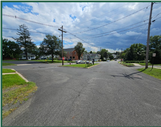
Figure 53. Looking to Main St. from Washington.
