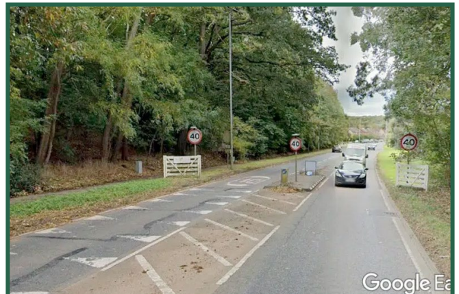
Figure 56. "Gateway Treatment" in rural England.
