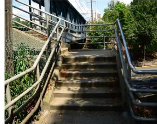
STAIRS FROM PARKING LOT 6 WALKWAY TO NEW YORK-BOUND PLATFORM
