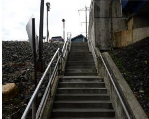
STAIRS FROM MAIN STREET SIDEWALK TO STATION PLATFORM AT PARKING LOT 2
