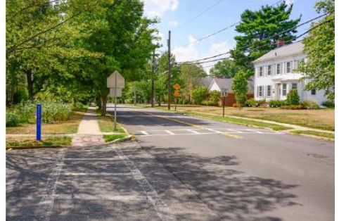
INTERSECTION OF WOODBRIDGE AVENUE AND BOUNTY STREET
