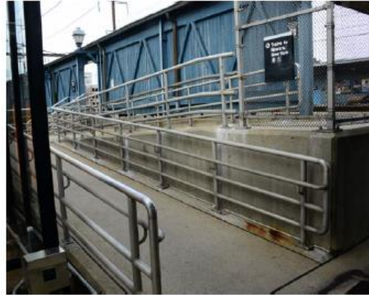
RAMP TO STATION PLATFORM IN PARKING LOT 1
