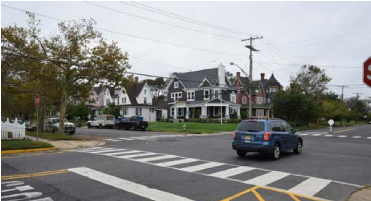
(Top) The intersection lacks ADA accommodations at all four crossings. (Bottom) Because cars and trucks park at the intersection, drivers are forced to inch out into the roadway to look for oncoming traffic.
