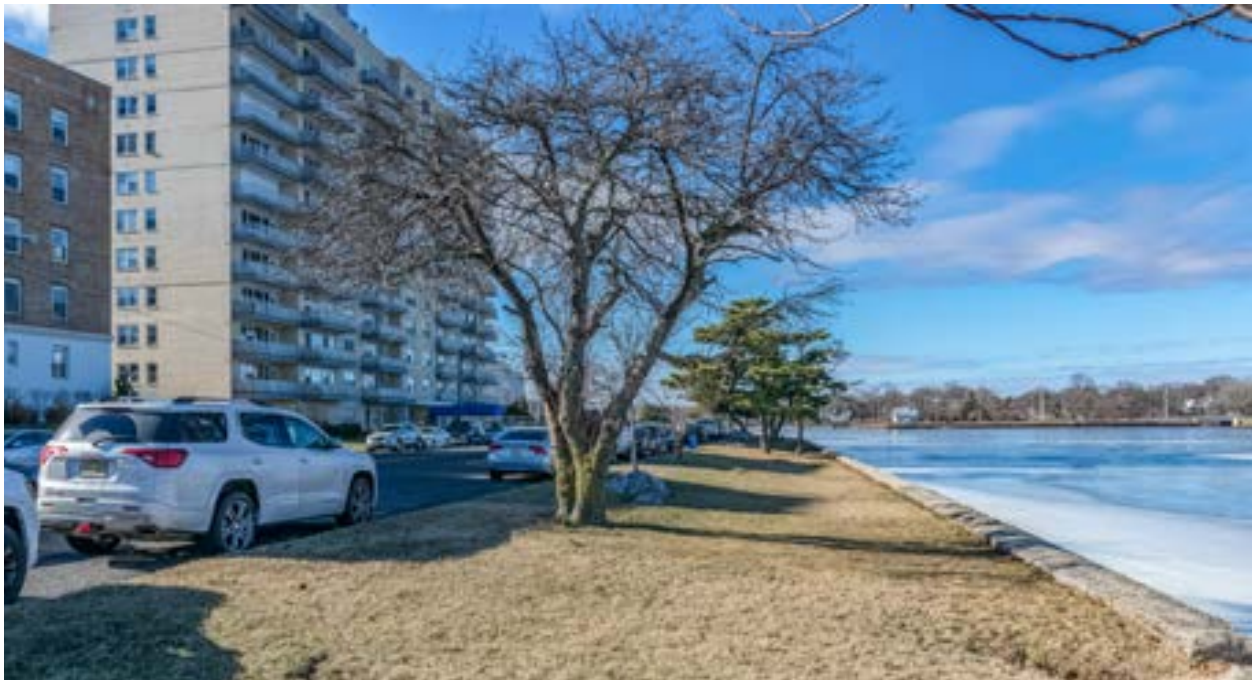
(Top) The northbound approach to Deal Lake Dr is excessively wide, resulting in fast turning vehicles and a challenging pedestrian crossing experience. (Bottom) A new sidewalk or shared-use path should be considered for the existing sidewalk gap on the north side of Deal Lake Dr
