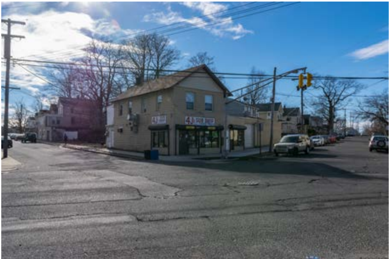
(Top) Vehicles blocking the crosswalk, rendering them ADA inaccessible. (Bottom) The intersection lacks crosswalks and ADA curb ramps
