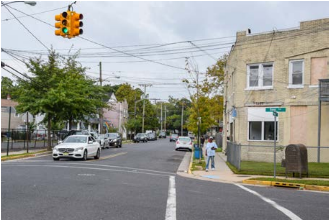
(Top) Vehicles frequently park at the intersection, compromising visibility for all intersection users. (Bottom) The intersection lacks pedestrian signals and highly visible crosswalks
