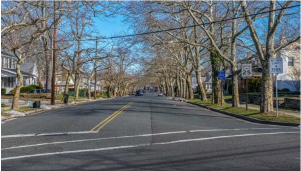
(Top) Existing intersection lacks individual curb ramps for each crossing and truncated dome pads. (Bottom) Existing crosswalks are not highly visible to motorists along 3rd Ave.
