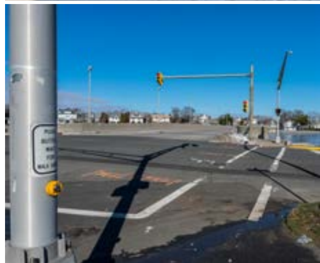
(Top) Signalized intersection lacking pedestrian signals at Asbury Ave & Church St/Pine St. (Bottom) Pedestrian signal at Park Ave & Deal Lake Dr (NJ 71) with pedestrian actuation. Ideally, the signal should have a dedicated pedestrian signal without the need for actuation.
