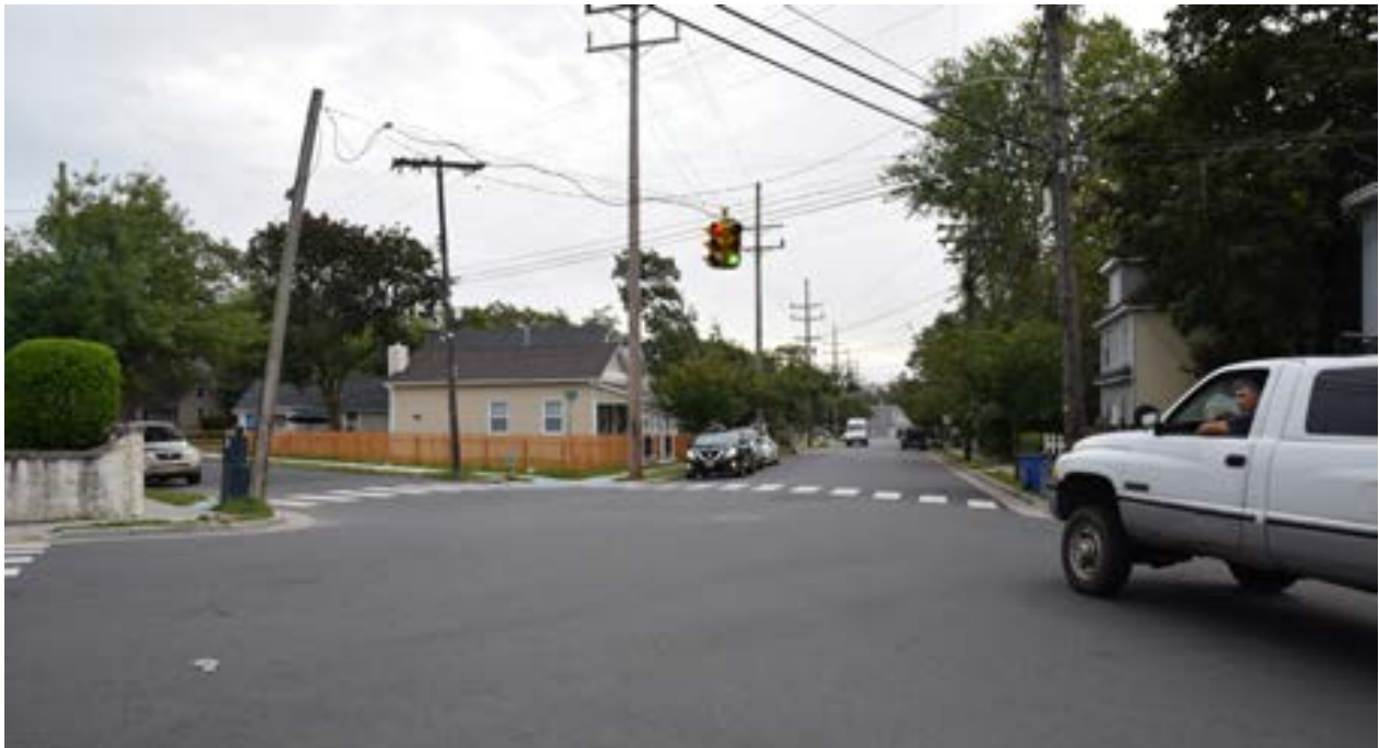
(Top) The intersection pedestrian signals. (Bottom) Due to a lack of centerlines and stop bars at the intersections, vehicles often stop well into the intersection
