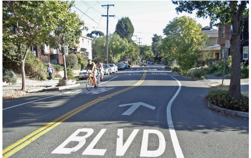
Example of a bicycle boulevard in Berkeley, CA that shows pavement markings and a chicane in the foreground, and a speed hump in the background. (Source: Flickr /Payton Chung)
