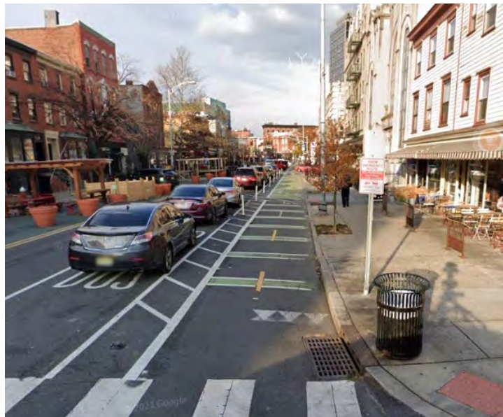
Physical barriers in this example protect the bicycle lane from adjacent vehicular traffic.
