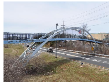
Grade separated crossing of US Route 22 in Bridgewater, NJ
