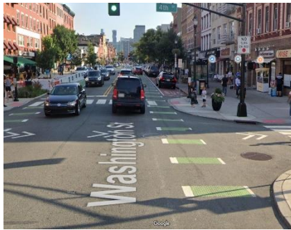
Pavement markings through intersection, Hoboken, NJ (Source: Google Streetview)
