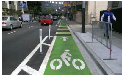
Picture of a buffered bicycle lane that is striped with paint on the street and is separated from motorized traffic by vertical elements, such as bollards (sturdy, short, vertical posts) or curbing (edge of a raised sidewalk). Source: NACTO
