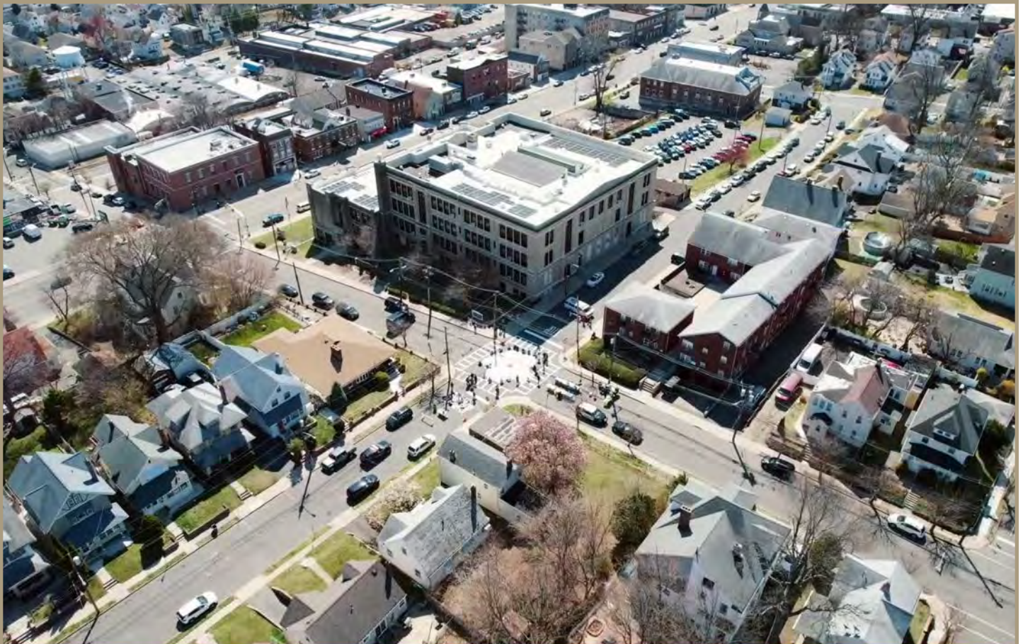
Figure 2. Aerial view of Belleville Middle School during the installation of the demonstration project.
