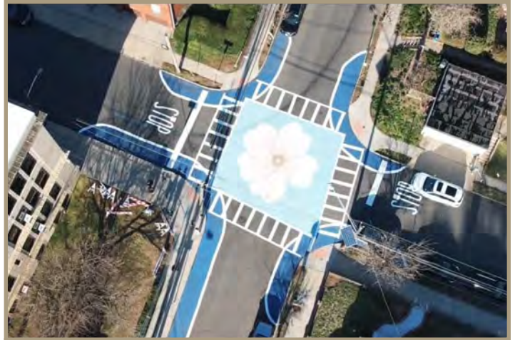
Figure 32. Installation as seen from above.
