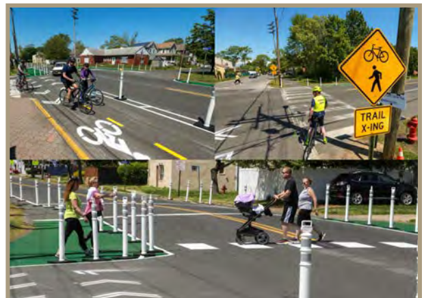
Figure 12. Bicyclists navigating the temporary on-road bicycle path in Keyport, NJ. Photos by NJTPA.
