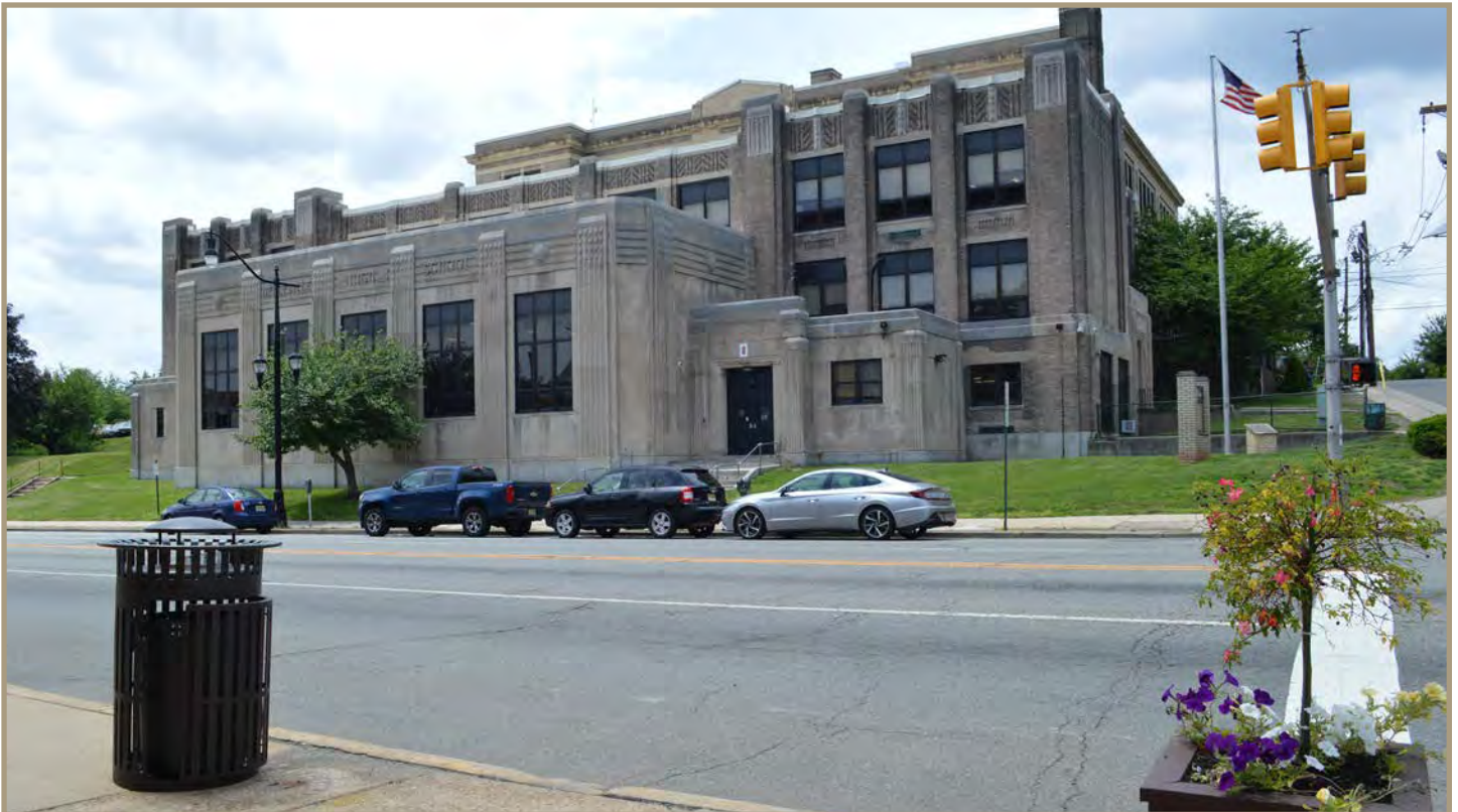
Figure 1. Belleville Middle School, as seen from Washington Street.
