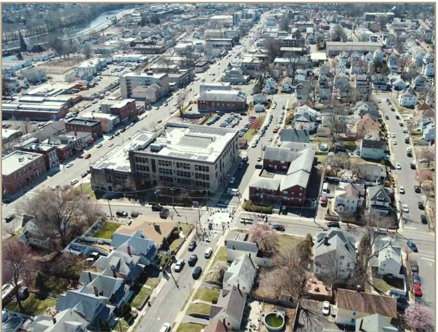
Figure 37. Belleville Middle School and surrounding neighborhood during the installation.
