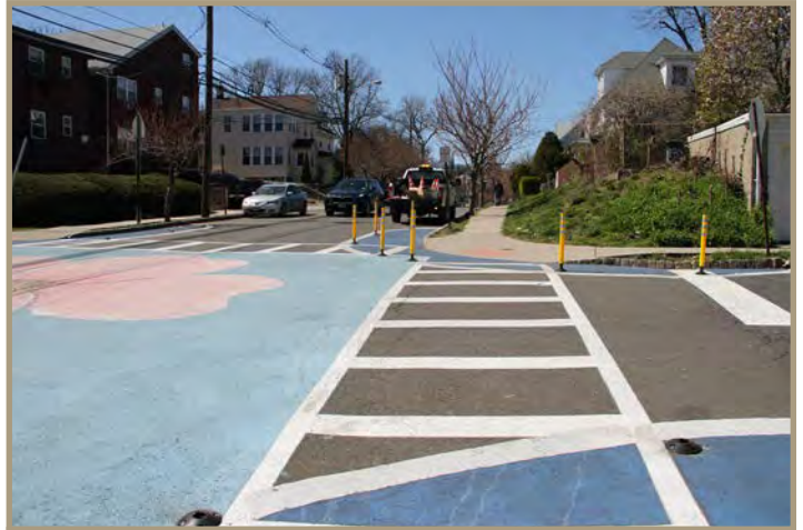
Figure 34. Addition of vertical delineators on April 10, 2023.
