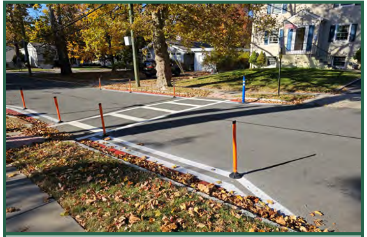
Figure 43. Curb extensions created with paint.
