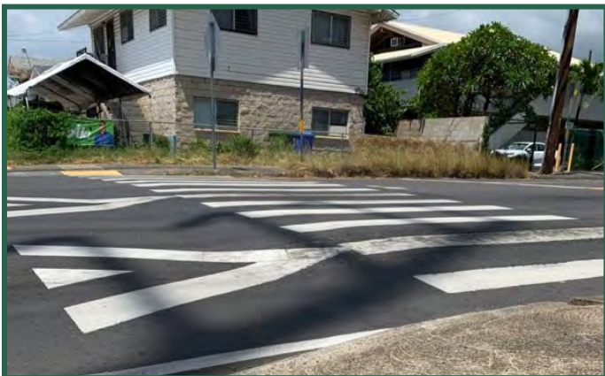
Figure 40. An example of a raised crosswalk.
