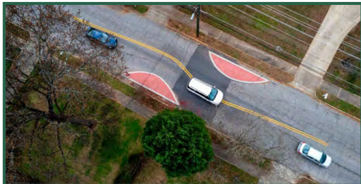
Figure 39. A permanent chicane example located at 3113 Brentwood Road, Raleigh, North Carolina.
