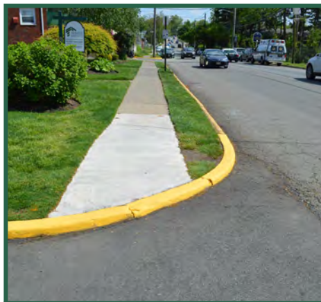
Figure 67. Additional missing curb ramps.
