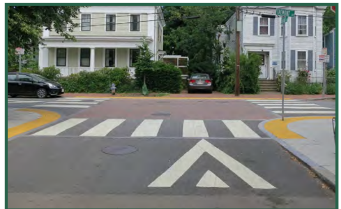
Figure 73. Raised intersection in Cambridge, MA.
