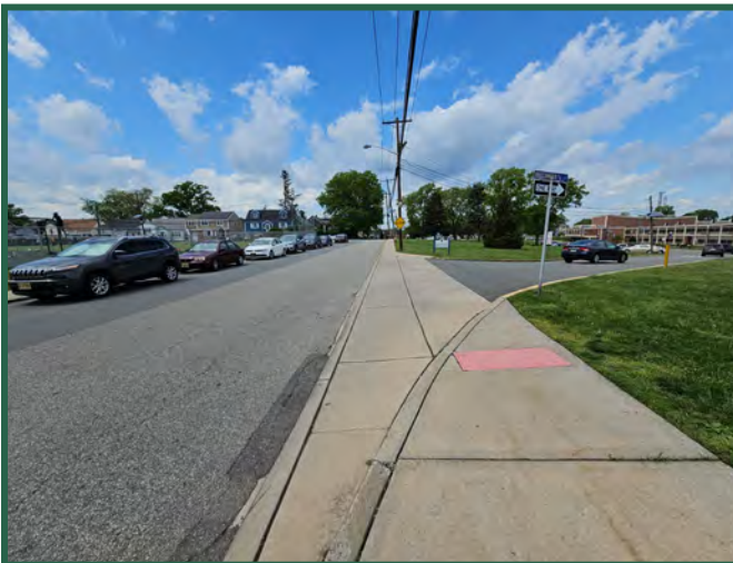
Figure 50. The extremely wide turning radius into school driveway is larger than needed for school buses.
