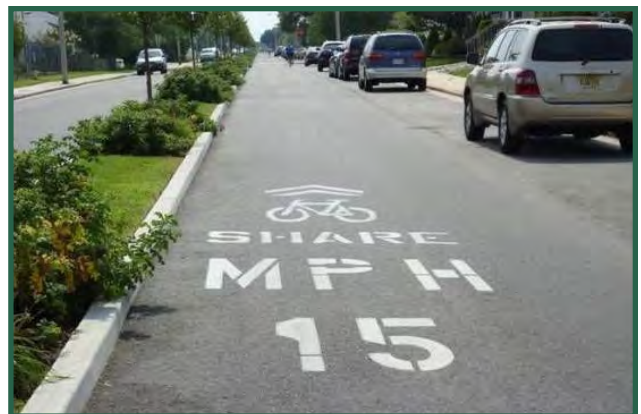
Figure 34. Pavement markings for a bicycle boulevard in Ocean City, New Jersey.
