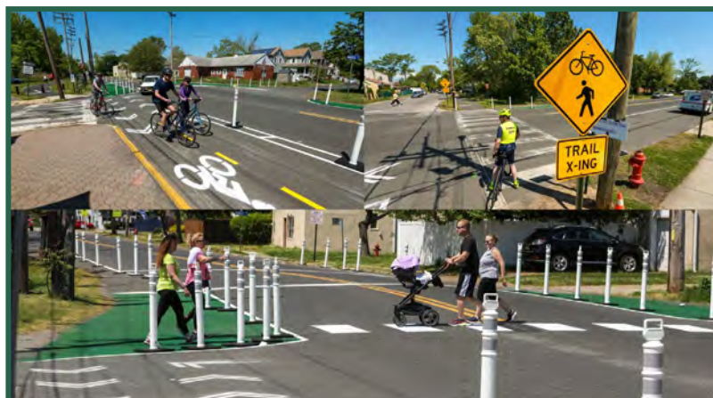
Figure 14. Bicyclists navigating the temporary on-road bicycle lane in Keyport, NJ. Photos by NJTPA.
