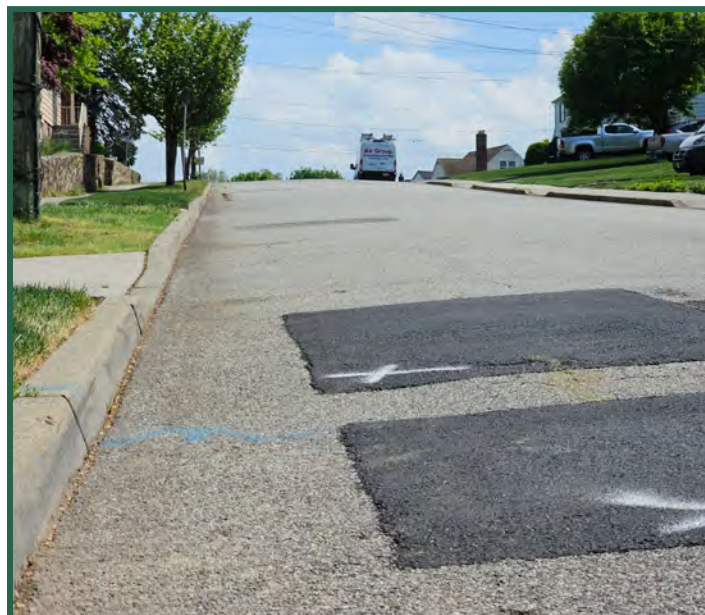
Figure 46. Looking south on Division Avenue where the roadway crests.
