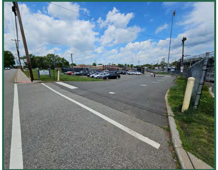
Figure 49. Austin Street/driveway entrance is wider than needed for vehicles, encouraging higher speeds.
