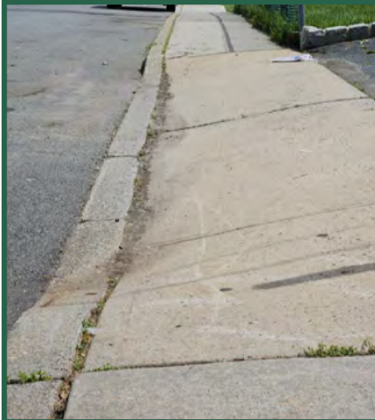
Figure 76. Sloped sidewalk at driveway.
