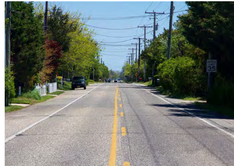
Sunset Boulevard, looking west at West Drive
