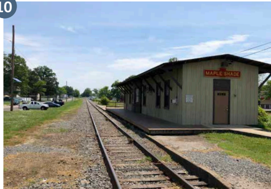
Maple Shade Station at N. Forklandng Road (view east).
