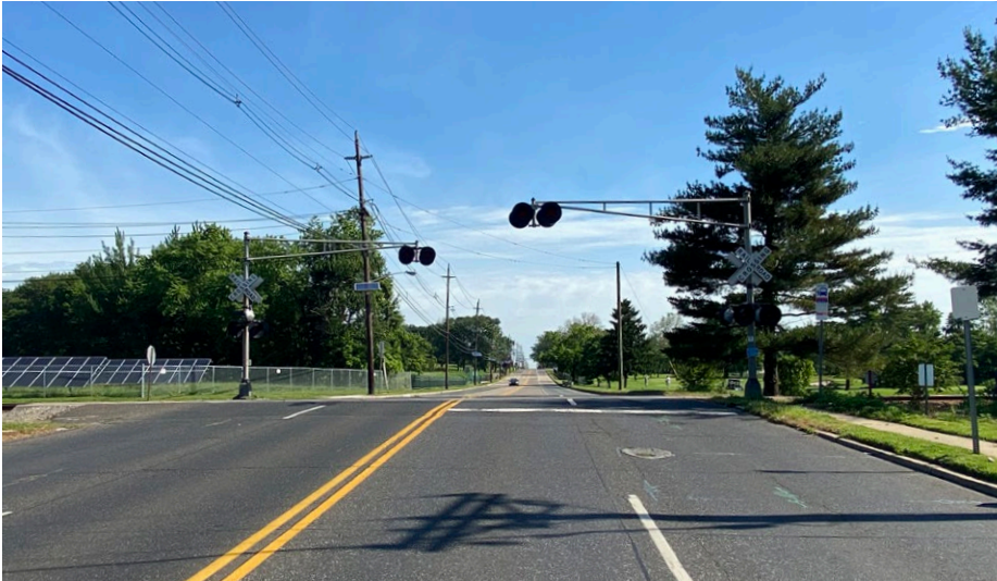
Pemberton Secondary crossing at Haddonfield Road (CR-644), view north.
