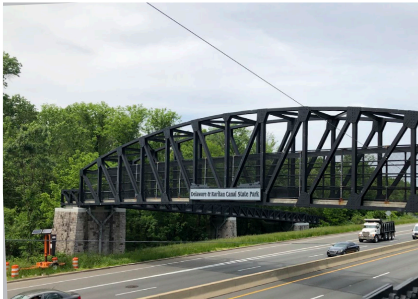
Example of a trail overpass at Delaware & Raritan Canal State Park, crossing US Route 1 in Lawrence Township, NJ.
