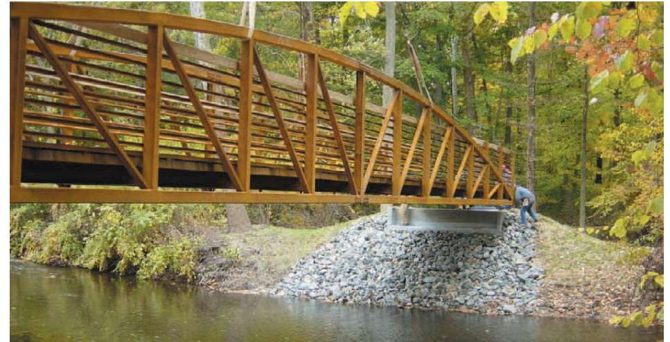
Example of a prefabricated bridge over the Whippany River, part of Patriots Path in Hanover Township, NJ (±75 foot span)
