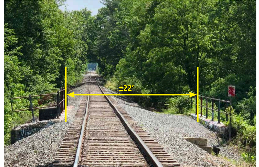
South Branch Pennsauken Creek Double Arch Culvert (view east)
