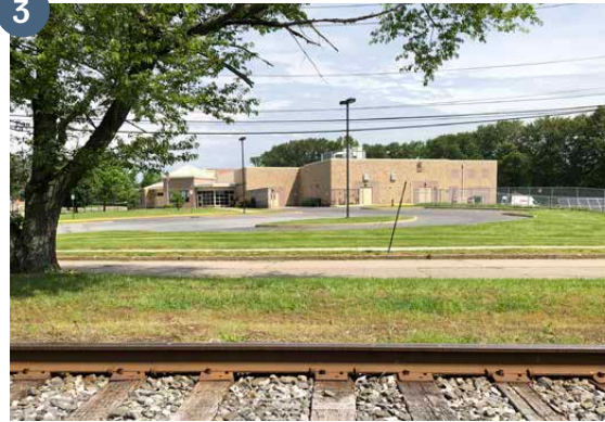
3 View north to Fine Elementary School near Haddonfield Road in Pennsauken.
