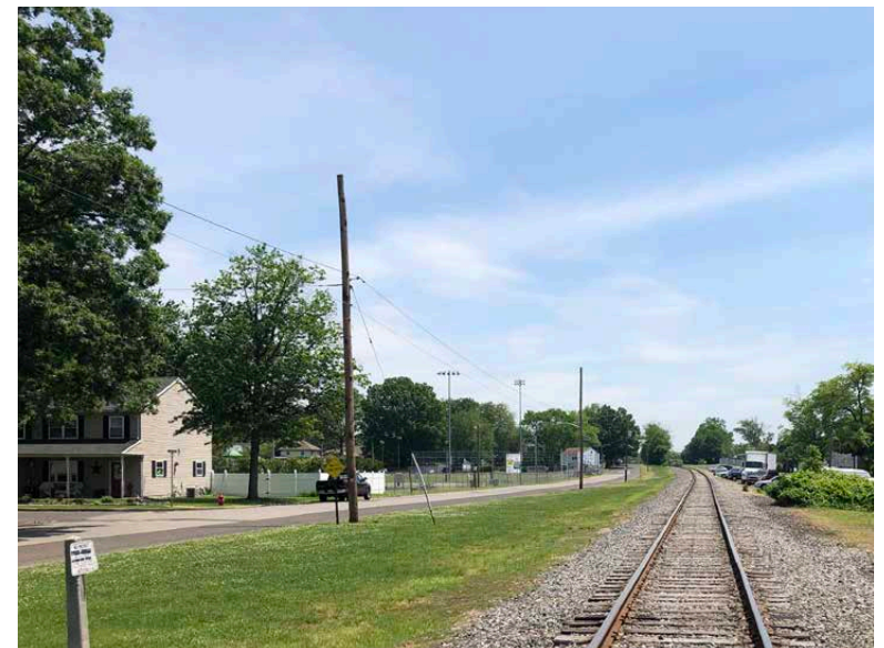
Utility poles along Broadway (northern edge of right-of-way) in Maple Shade.
