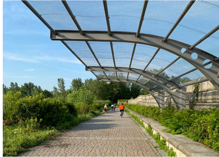
Example of a golf hazard mitigation structure installed to protect trail users and preserve waterfront views along the Hudson River Waterfront Walkway at Liberty State Park in Jersey City, NJ.
