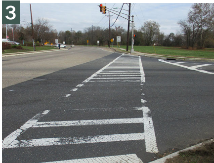
Route 130 NB view across Jacksonville Road (CR 670)
