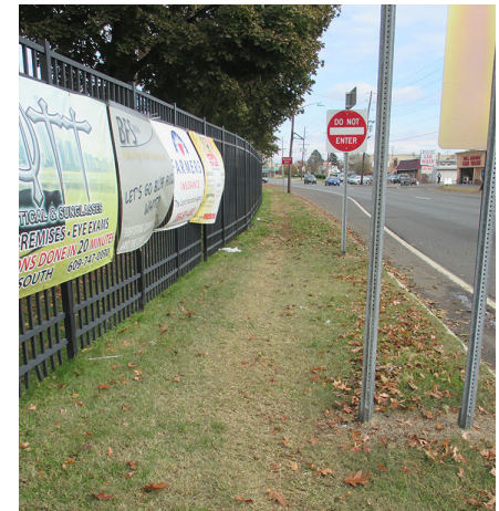
Missing sidewalk near Wilbur Watts School, Burlington City, NJ
