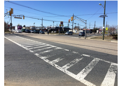
Example of long crossing
