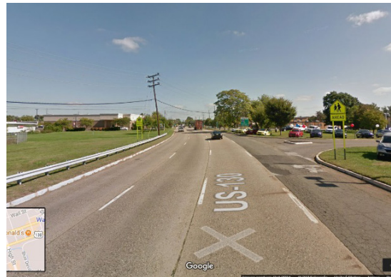
Route 130 NB (between Wood Street and High Street) before road diet
