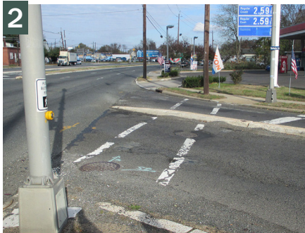
Route 130 NB view across Salem Road
