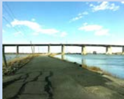
Access Road to Boonton / Newark Industrial Tract, Kearny, NJ
