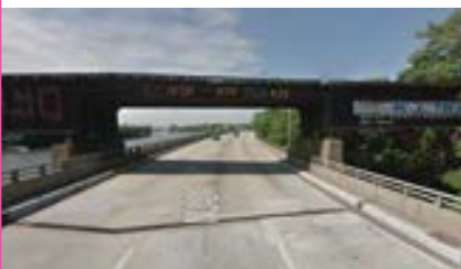
Boonton Line: Route 21 (Passaic River)
