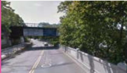
Boonton Line at Passaic Avenue, Kearny
