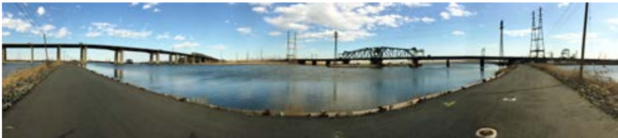
Photo: Access roads to the Boonton and Newark Industrial Tract
