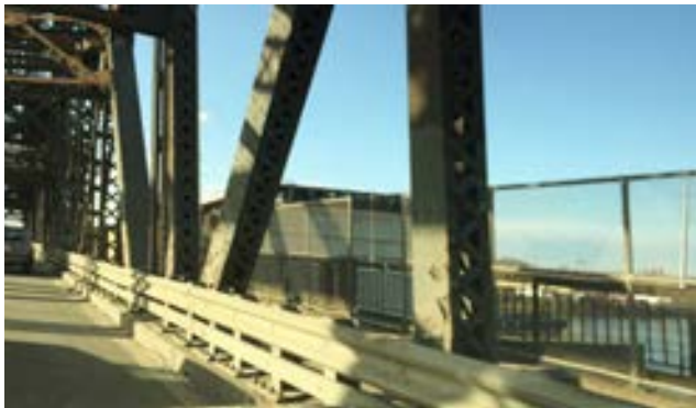
Existing Wittpenn Bridge, Source: NV5, Inc
