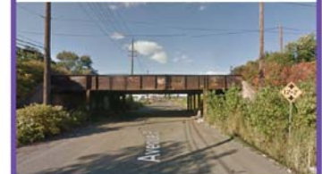
Railroad Corridor & Avenue P, Newark
