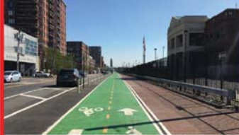
Observer Hwy, 2-way Protected Bike lane & Pedestrian Walkway, Hoboken
