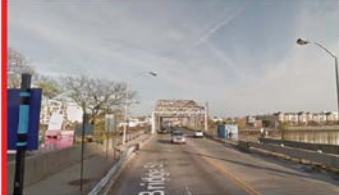
Bridge Street Bridge, Newark
