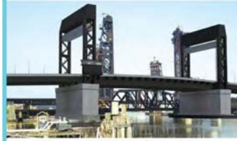
WittPenn Bridge, Hackensack River Under construction
