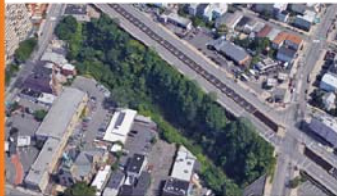
Bergen Arches Aerial View, Jersey City
