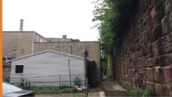
6th Street Embankment, Jersey City
