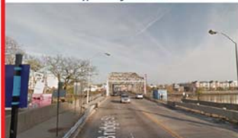
Bridge Street Bridge, Newark
