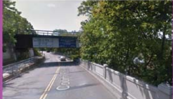
Boonton Line at Passaic Avenue, Kearny
