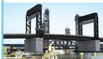
Wittpenn Bridge, Hackensack River Under construction
