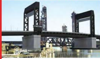
WittPenn Bridge, Hackensack River Under construction
