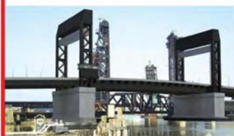
Wittpenn Bridge, Hackensack River Under construction
