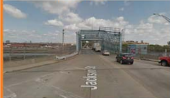
Frank Rodgers Bridge, Newark/Harrison
