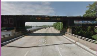
Boonton Line: Route 21 (Passaic River)
