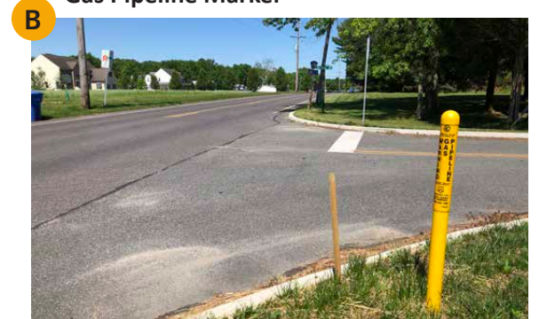
Gas Pipeline Marker
