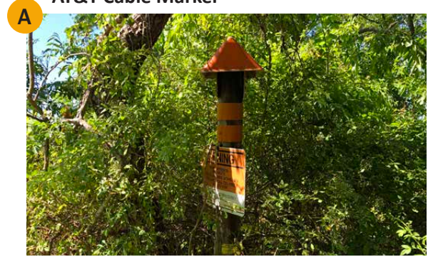
AT&T Cable Marker
