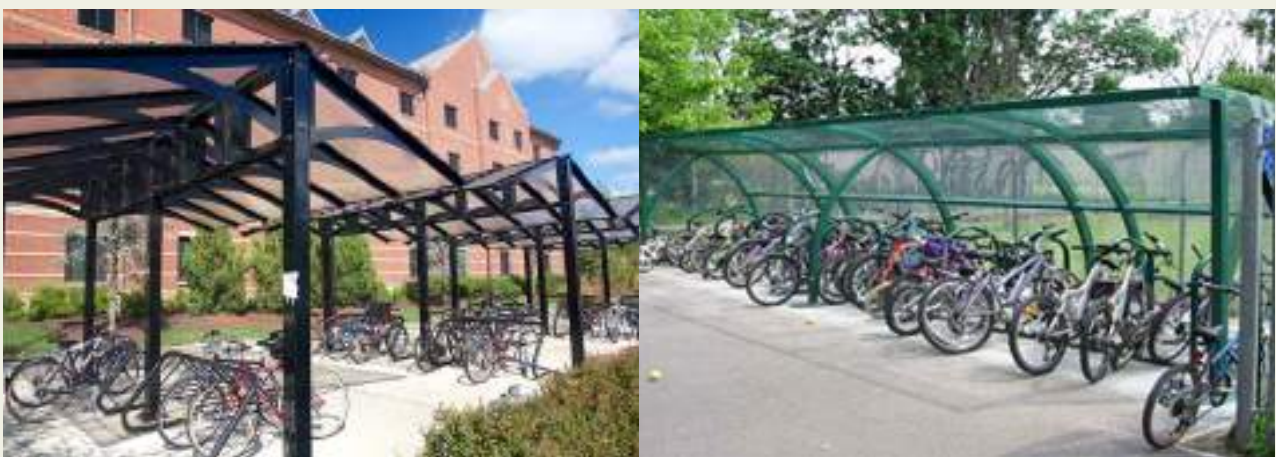
Examples of covered bicycle parking at Rutgers University (left) and a school in London, UK (right, source: guide.saferoutesinfo.org )
