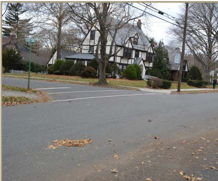
Figure 18. Crosswalks across Hamilton Avenue are absent at the various T-intersections, (looking north on Hamilton Avenue).
