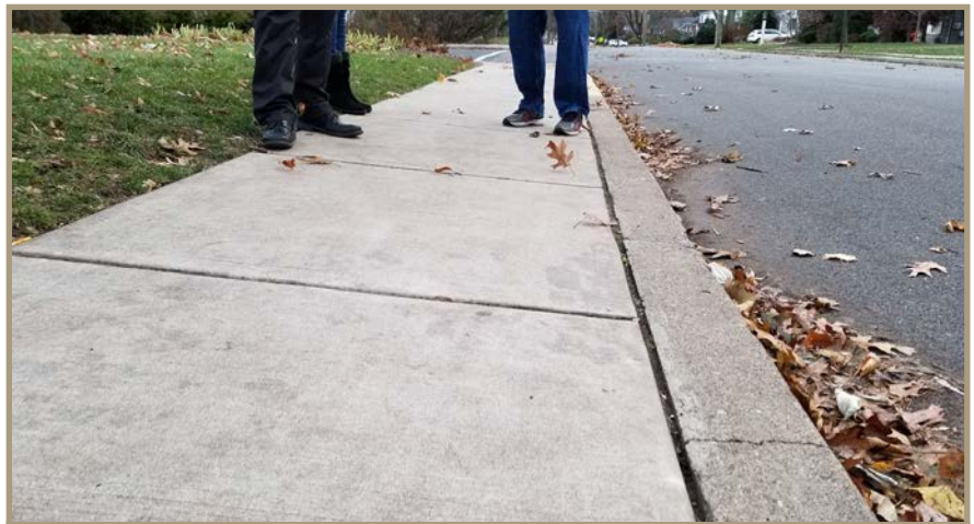
Figure 17. Sidewalk sloped towards roadway.
