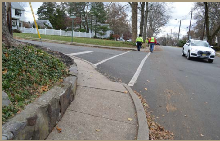
Figure 38. At Gramercy Place, the sidewalk narrows, there is a strong cross-slope, the corner ramp is not ADA compliant, and the wide turning radius encourages faster vehicle speeds.
