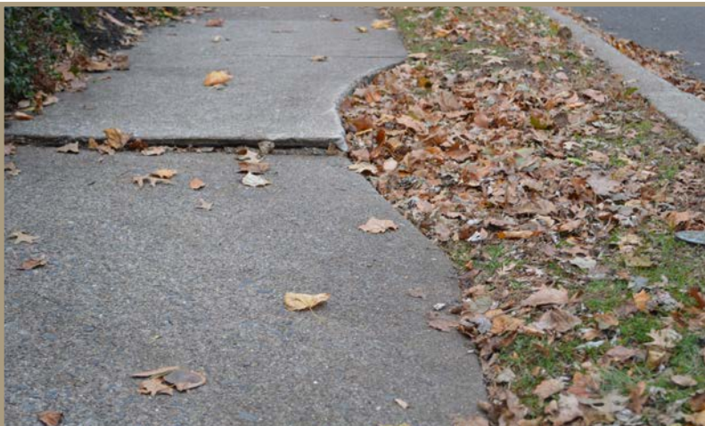
Figure 14. The sidewalk frequently narrows where mature trees once stood. The roots of those trees have raised the sidewalks at some locations.
