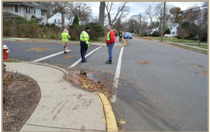
Figure 39. The curb ramp at Emerson Road accumulates debris, and is not ADA compliant. There is no marked crosswalk across Hamilton Avenue.
