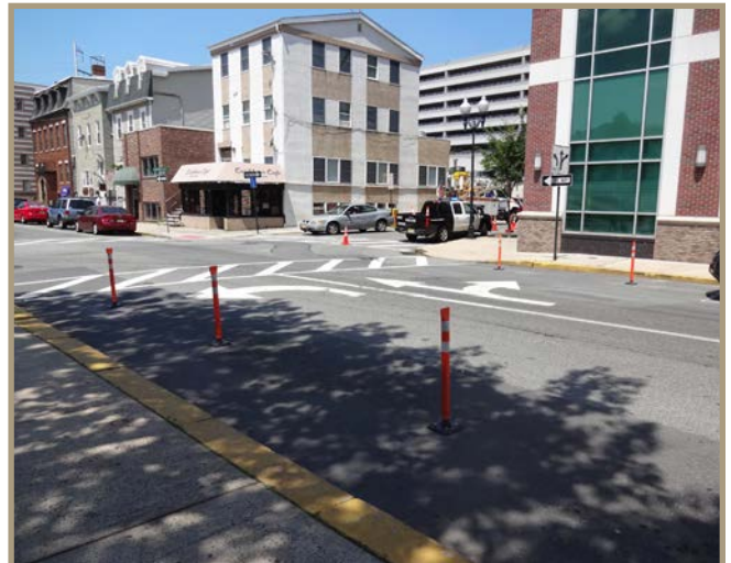
Figure 56. New Brunswick, NJ, uses plastic bollards to prevent illegal parking near intersections. After a successful trial at one intersection, the city has added them throughout the city.
