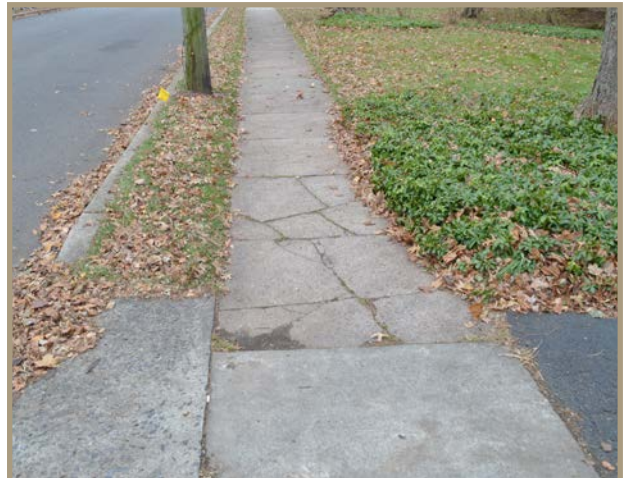
Figure 15. The corridor has continuous sidewalks on both sides, although cracking is apparent in parts.
