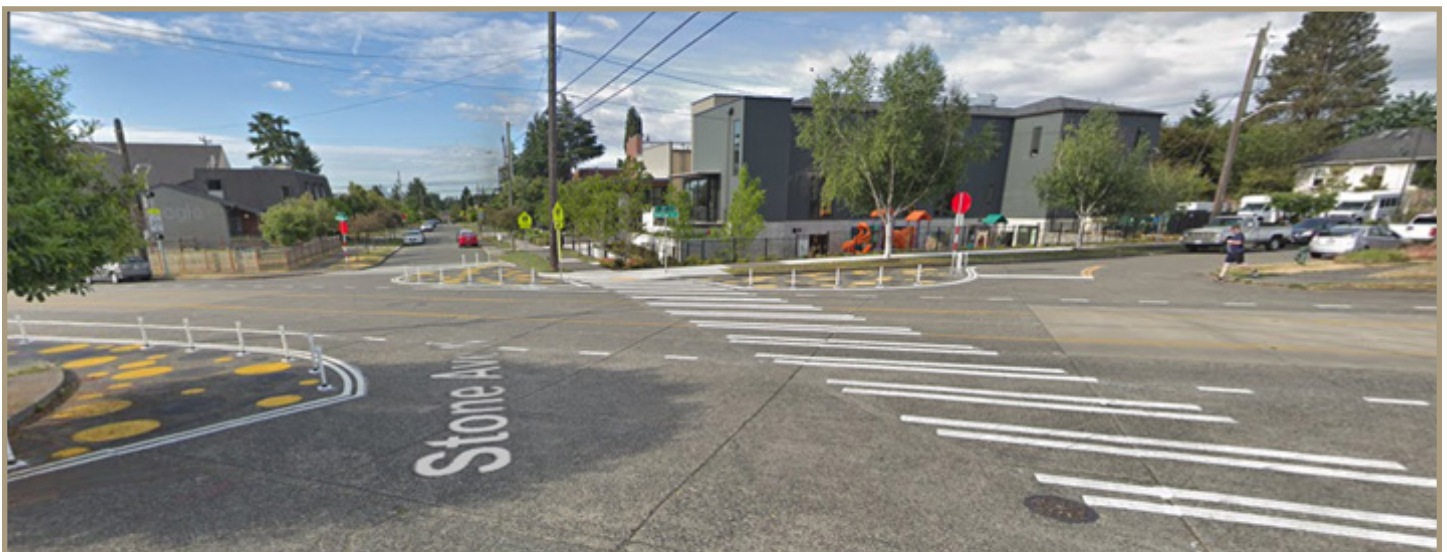
Figure 57. Curb extensions using plastic bollards and paint have been used in Seattle to realign confusing intersections, slow traffic, and add new pedestrian crossings.
