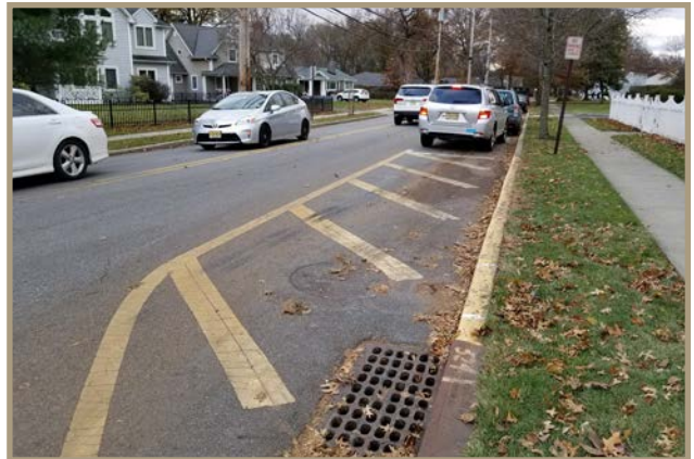
Figure 41. The crosshatch striping on Harristown Road effectively deters illegal parking (looking west).
