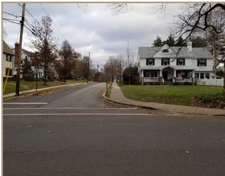
Figure 20. Wide turn radius at various intersections.
