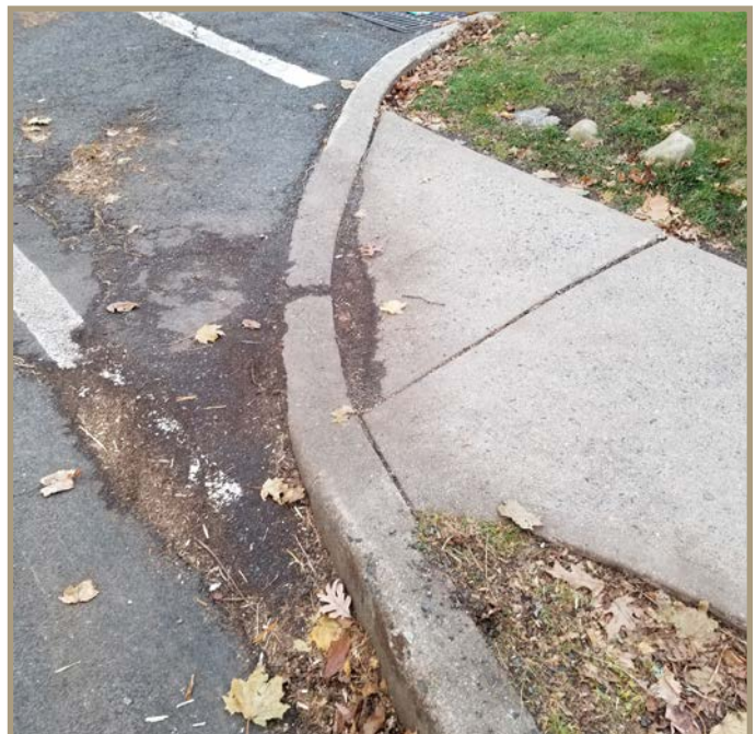
Figure 21. Ramps not ADA compliant along corridor.
