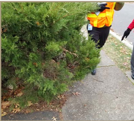
Figure 16. Sidewalk blocked by vegetation.
