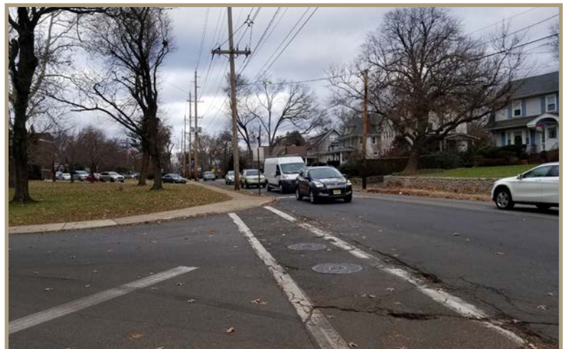
Figure 32. Drivers did not block the intersection when observed during the audit (looking northeast).
