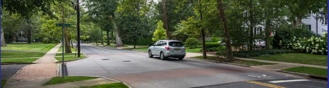
Raised intersections help both calm traffic and enhance pedestrian crossings.
