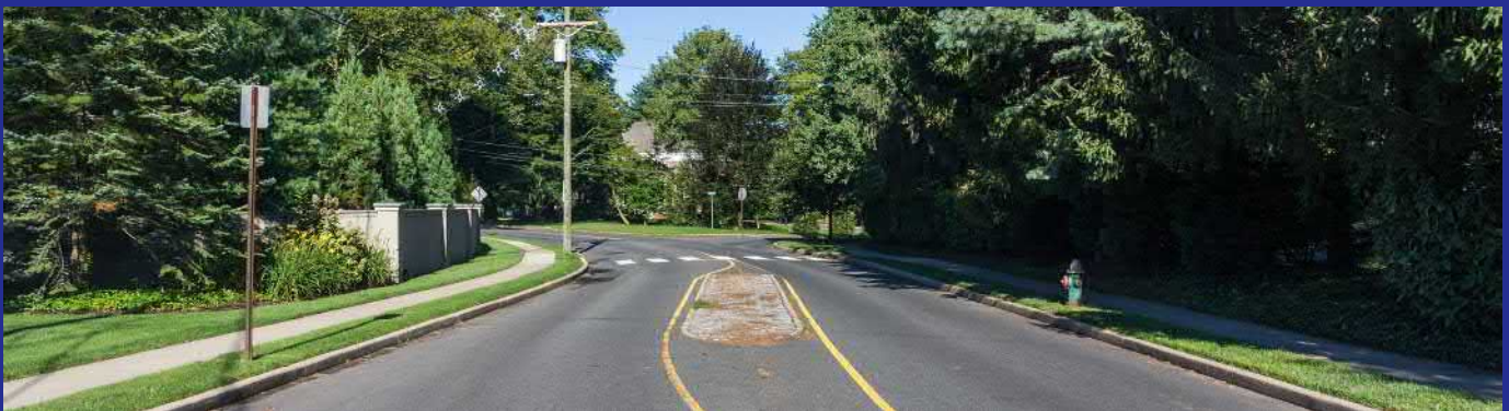
Median islands calm traffic by narrowing the travel lane. Median islands are a versatile treatment, ranging from a cobblestone island that can be easily mounted by vehicles (as shown above) to a raised curb island with street trees or other features.
