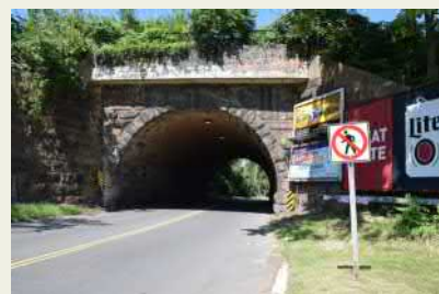
River Rd underpass of NEC Tracks
