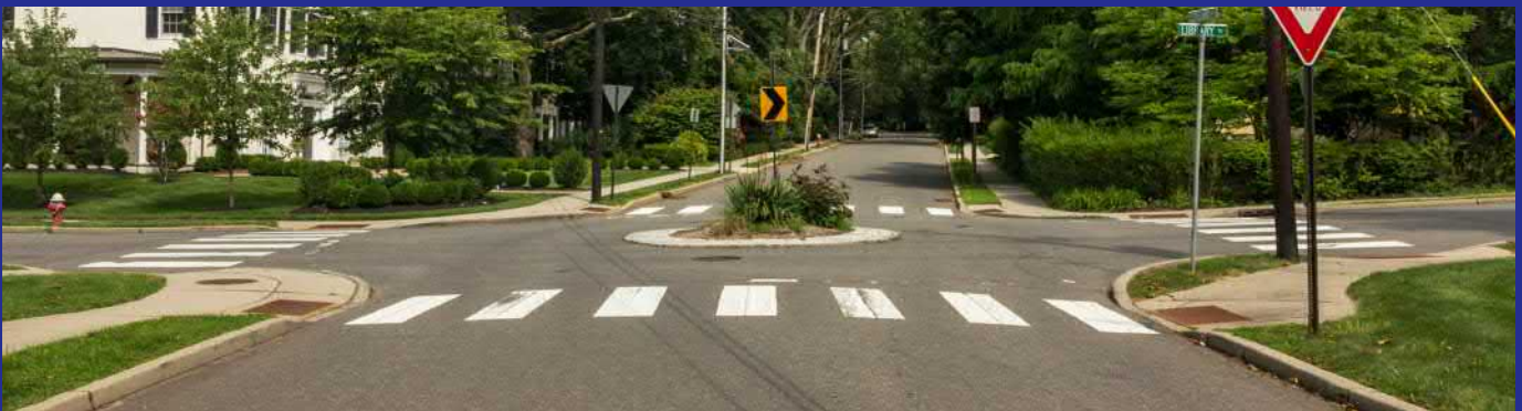
Neighborhood roundabouts, which also narrow travel lanes and tighten turning radii at intersections to reduce traffic speeds. Other treatments used with similar impacts include neckdowns (midblock curb extensions to narrow the roadway) and speed humps.
