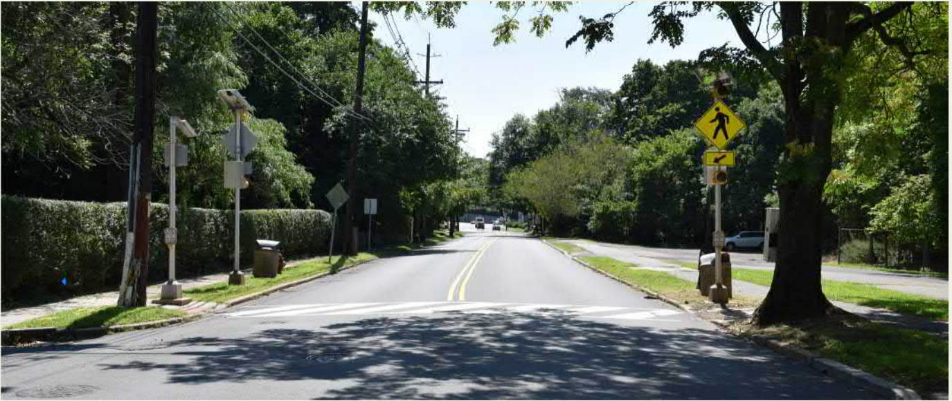
RRFBs at River Rd at Harrison Ave
