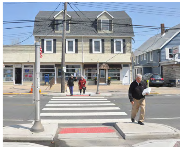
Mid-block Crossing with curb extension and signal actuation in Bayhead, NJ
