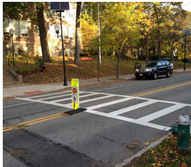
In-Street Pedestrian Crossing Sign in Montclair, NJ
