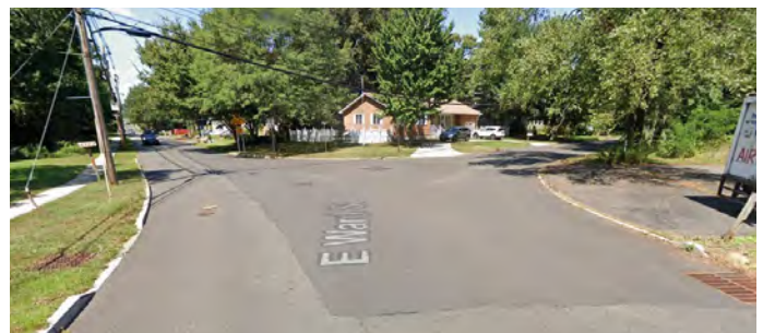
PHOTO: WIDE TURNING RADII FROM E WARD STREET ONTO MAXWELL AVENUE
