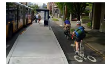
Floating Bus Island in Seattle, courtesy of NACTO Urban Street Design Guide
