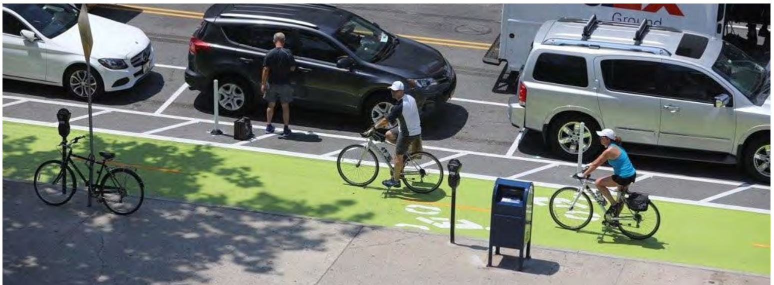
Protected Bicycle Lane (Grove Street)
