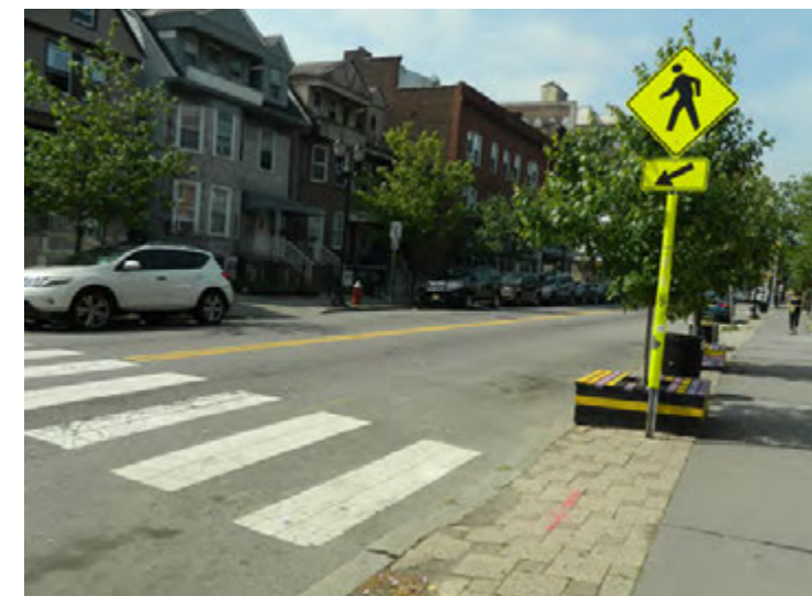
Marked Crosswalk in Jersey City
