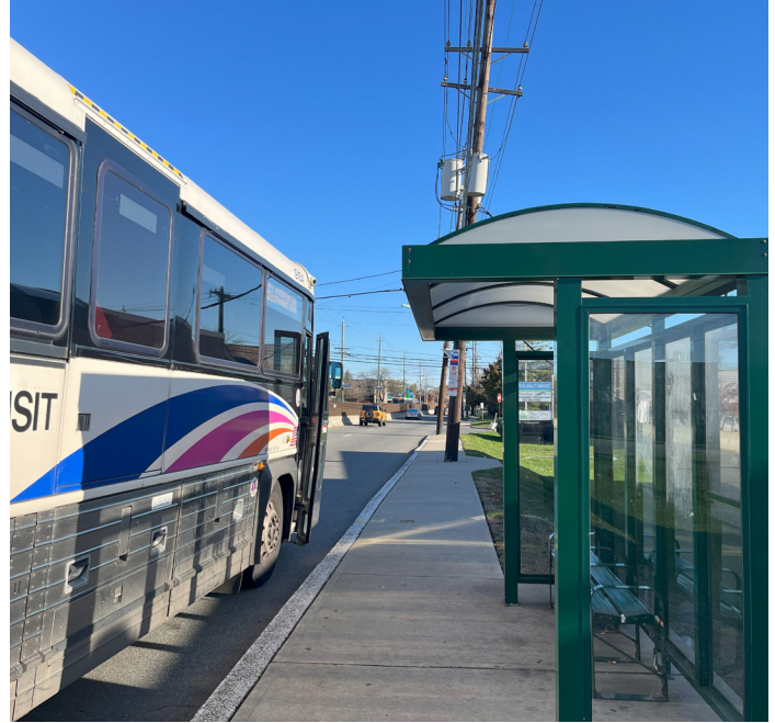
Figure 39 Bus stop located on the east side of Washington Avenue, north of Barell Avenue. Source: SGB, LLC
