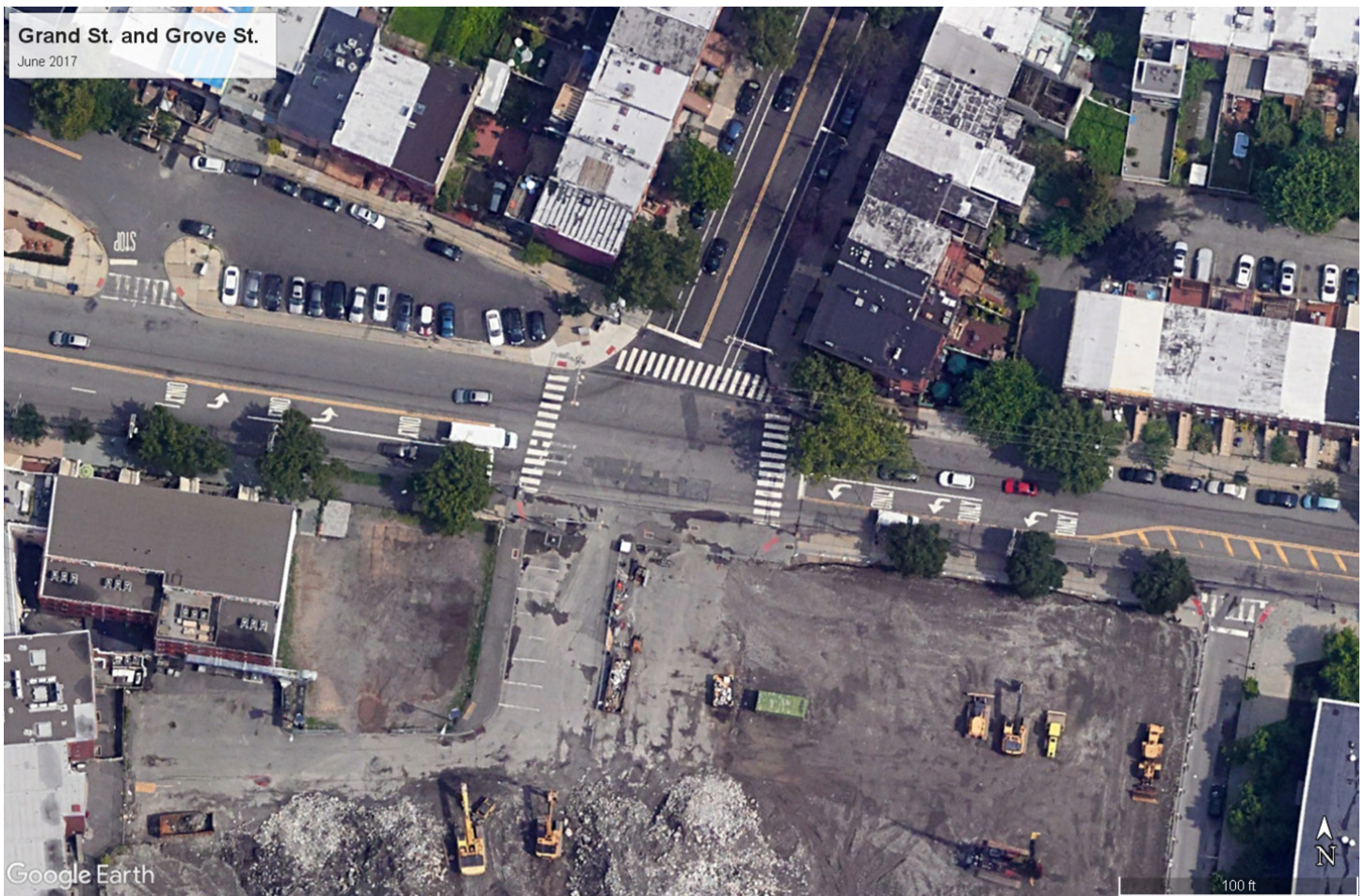
Figure 5 Aerial of Grand and Grove Streets intersection in June 2017, before countermeasure implementation. Source: Google
