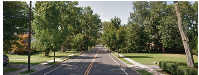
STREET VIEW (NORTHBOUND)
