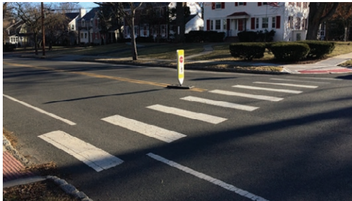
Example of high-visibility crosswalk striping on Prospect St Credit: NV5
