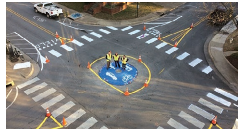
Temporary roundabout with striped curb extensions Credit: Snellville.org
