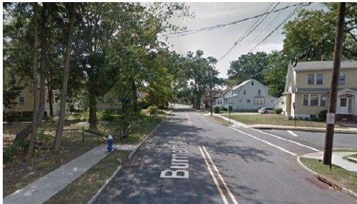
Missing curb ramp on Burnett Avenue Credit: Google Maps
