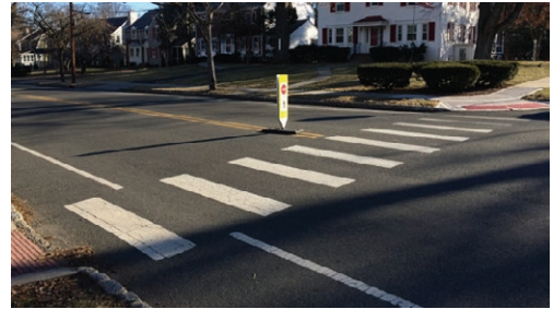
Example of high-visibility crosswalk striping on Prospect St Credit: NV5
