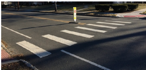
Example of high-visibility crosswalk striping on Prospect St Credit: NV5
