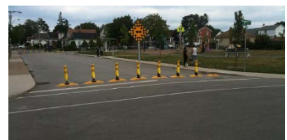
Temporary Street Closure Credit: Raisethehammer.org
