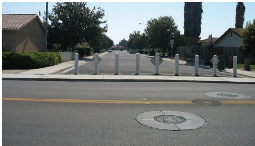
Example of permanent street closure in Stockton, CA Credit: Stockton.gov
