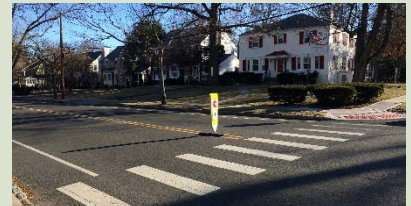
High-visibility crosswalk Credit: NV5
