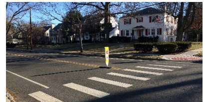
High-visibility crosswalk Credit: NV5
