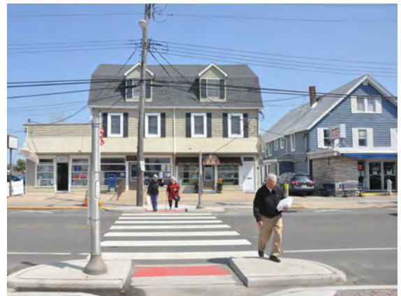
Mid-Block Crossing with curb extensions and signal actuation in Bayhead, NJ
