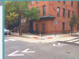
Low-Cost Curb Extensions and continuous bicycle markings, Hoboken, NJ
