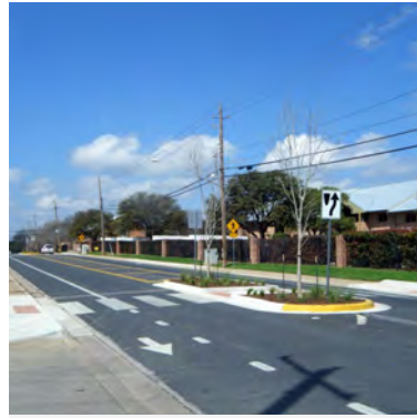
Planted median, Austin, TX Credit: NACTO
