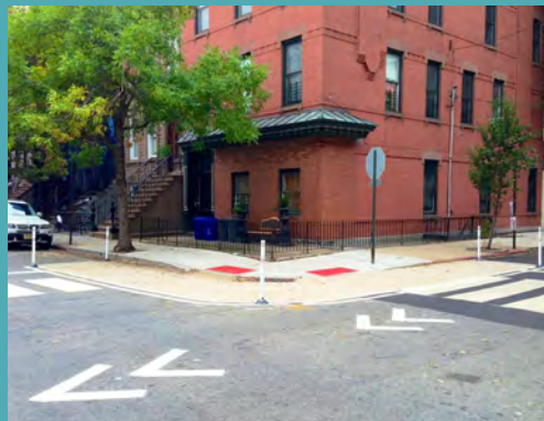
Low-Cost Curb Extensions and continuous bicycle markings, Hoboken, NJ
