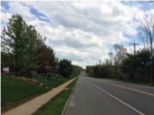
Wolfe Rd existing sidewalk
