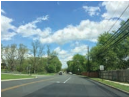
Flanders Bartley Rd looking east at Siemens
