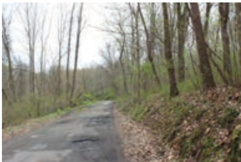
Waterloo Valley Rd
