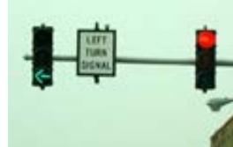
Protected Left Turn Phases Can reduce conflict between left-turning vehicles and greenway travelers
