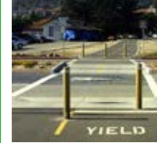
Bollards create a physical barrier to alert or slow control greenway users at roadway crossings and prevent unauthorized vehicle access. Bollards are highly configurable to a range of looks and finishes.
