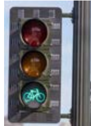
Bicycle (or standard) signal heads are oriented to greenway users and improve dedicated signal phasing applications
