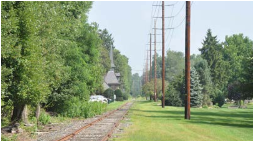
Example of overhead distribution lines on the east side of the study area right-of-way (view north toward Demarest Station).
