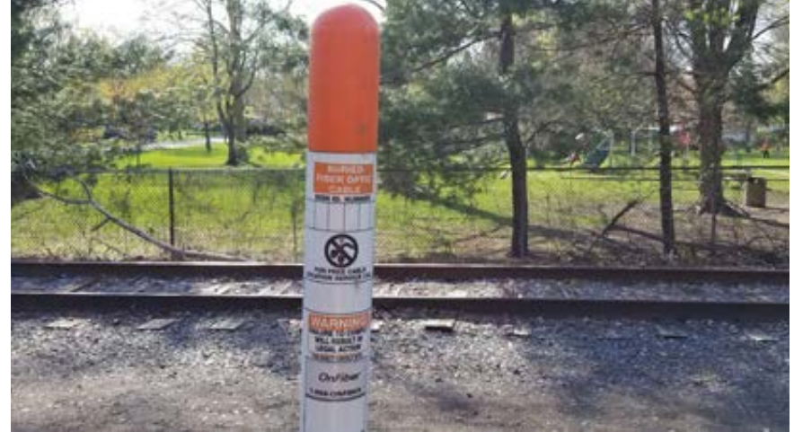
Example of a buried fiber optic cable marker in Dean Park in Tenafly.
