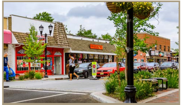
Figure 37. A raised midblock crossing with curb extensions, seating and plantings in Union Township, New Jersey. (Photo credit: Arterial LLC)
