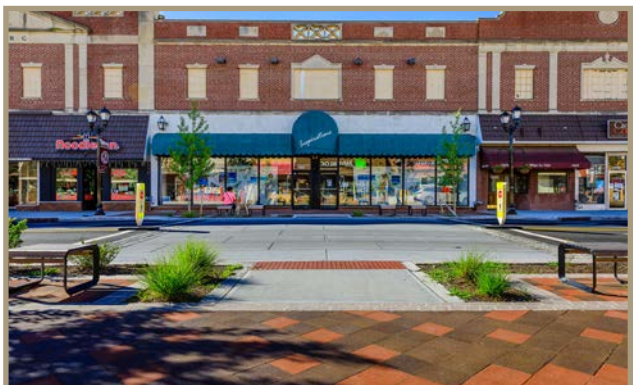
Figure 40. The mid-block crossing in Union Township, New Jersey, is at sidewalk level and provides ADA accommodations. (Photo credit: Arterial LLC)
