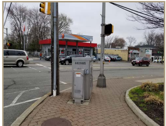
Figure 30. Access to the only ramp located at the southwest corner of the Lake Shore Drive intersection is constricted by the placement of a traffic signal controller box, pedestrian signal, and telephone pole.
