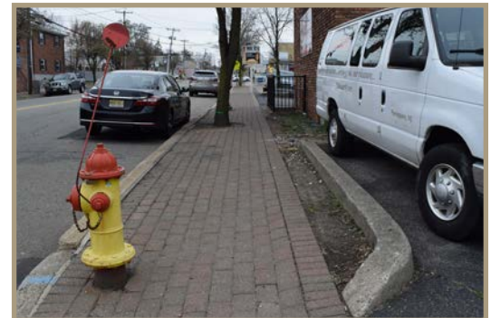
Figure 47. Sloping sidewalk and uncovered tree wells looking south on North Beverwyck Road, north of Lake Shore Drive.
