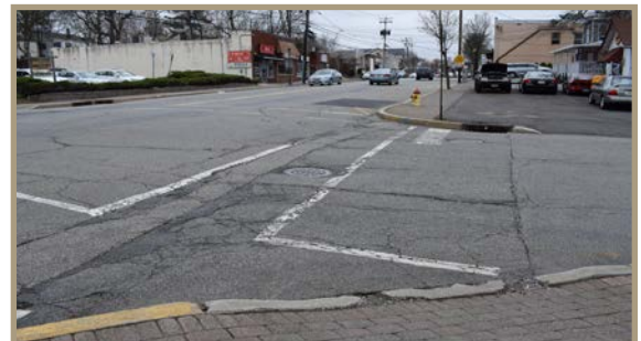
Figure 26. Missing curb ramp and steep, eroded ramp at the intersection of North Beverwyck Road and Minnehaha Boulevard, looking northward.
