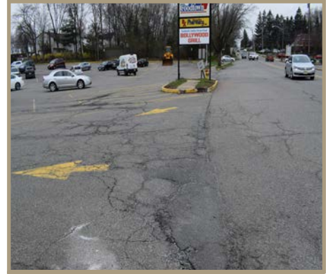
Figure 14. Missing sidewalks in front of Foodtown, looking south on North Beverwyck Road.
