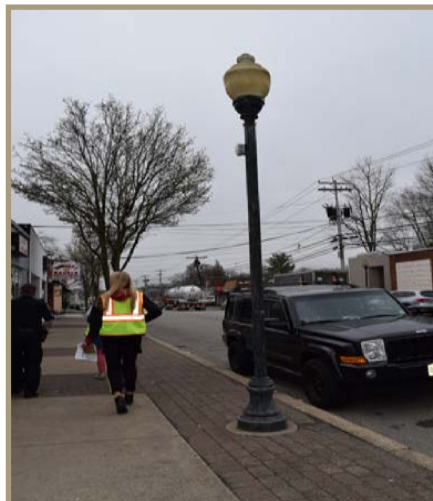
Figure 23. Pedestrian lighting that does not direct light onto the sidewalk, looking southward on North Beverwyck Road near the intersection of Hiawatha Boulevard.
