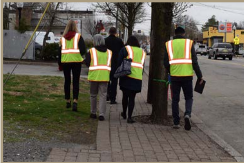
Figure 12. An uncovered tree well takes up most of the usable sidewalk space and uneven pavers create a hazard, looking northward on North Beverwyck Road, south of Lake Shore Drive.
